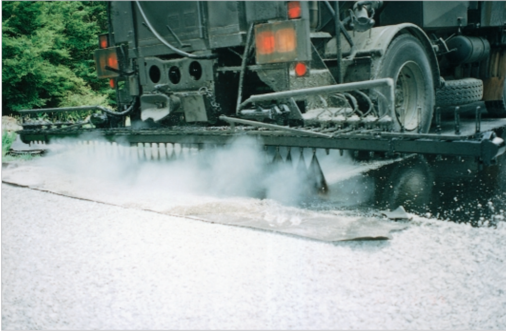
Figure 10-10 Use paper to make an accurate start line when starting a spray run.
