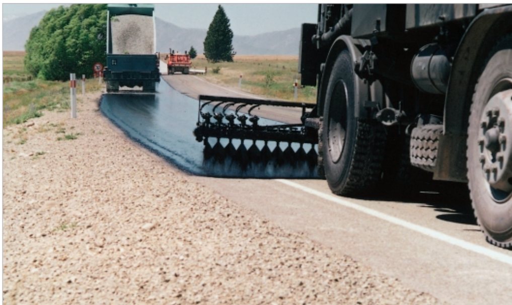
Figure 10-1 A sprayer in operation showing the spray fans. Note the different shape of the fan coming from the end nozzle. Photo courtesy of Lindsay Roundhill, Opus
