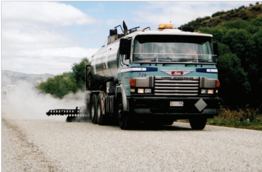
Figure 10-17 A bitumen distributor in action.
