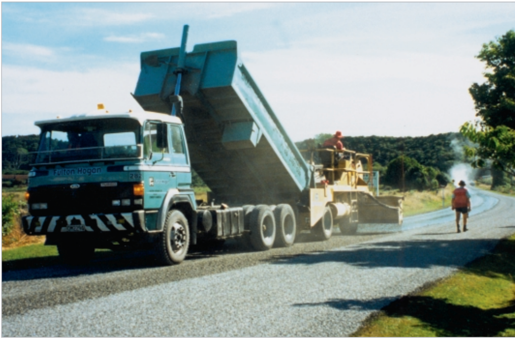
Figure 10-18 A truck supplying chip to a self-propelled chipspreader during a chipsealing operation. Photo courtesy of Les McKenzie, Opus
