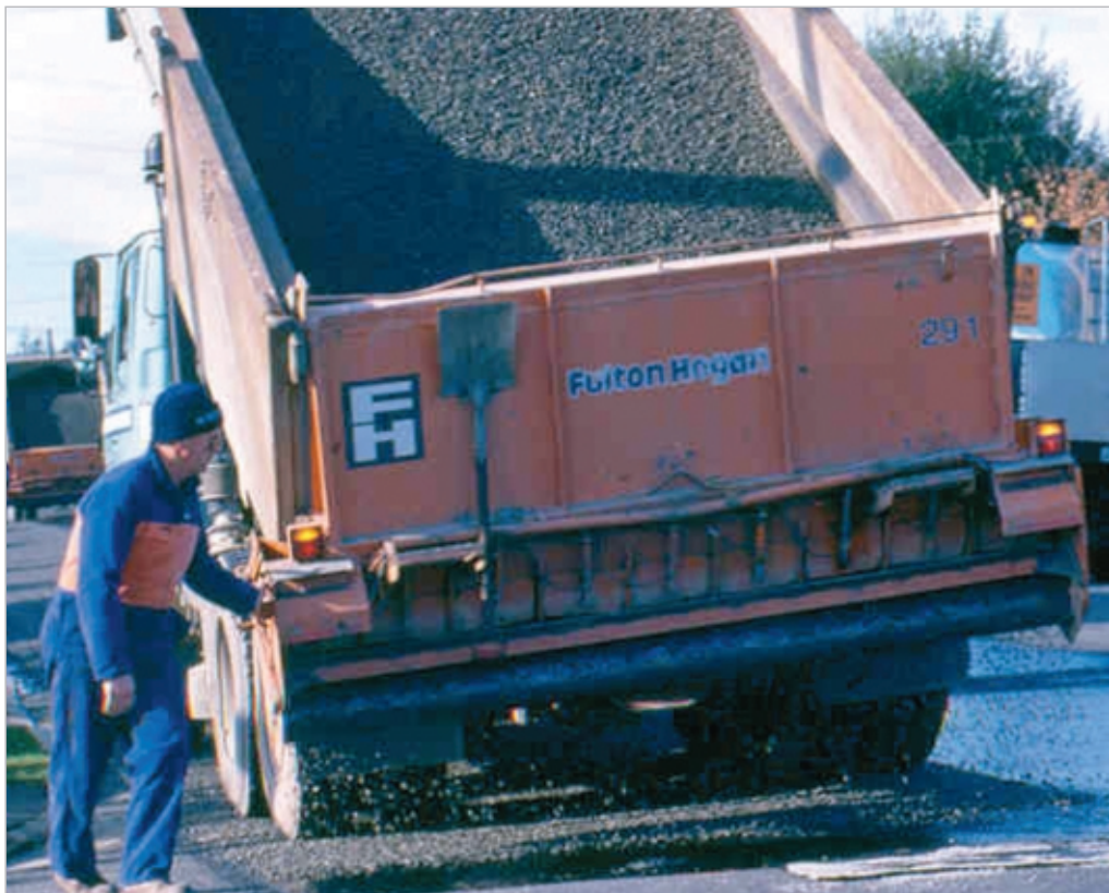
Figure 10-21 Procedure for calibrating chip spreading on paper.
