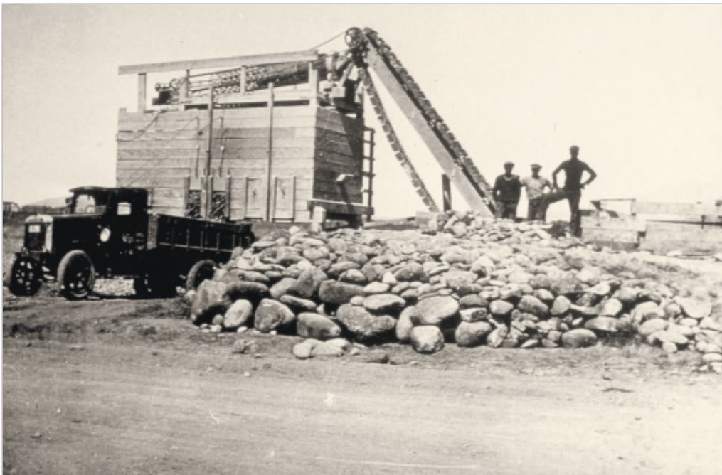
Figure 8-20 Screening aggregate for road use from a beach near Opunake, Taranaki, in the 1920s.
