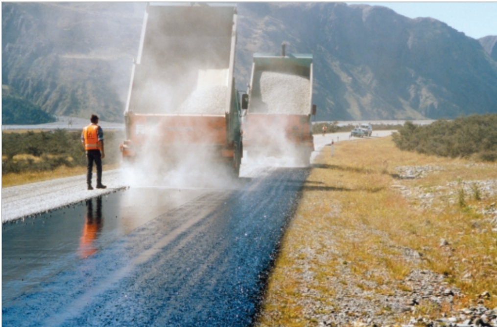
Figure 8-26 Clouds of dust when applying chips may indicate that they have low cleanness value. Photo courtesy of Les McKenzie, Opus
