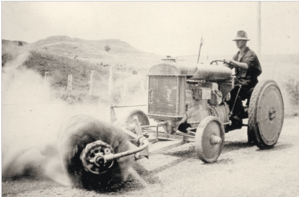
Figure 7-1 The basecourse for State Highway 2 in Cook County, Gisborne, was swept clear of loose aggregate and other detritus by this rotary broom mounted in front of a tractor (with solid wheels and tyres), in the 1920s.
