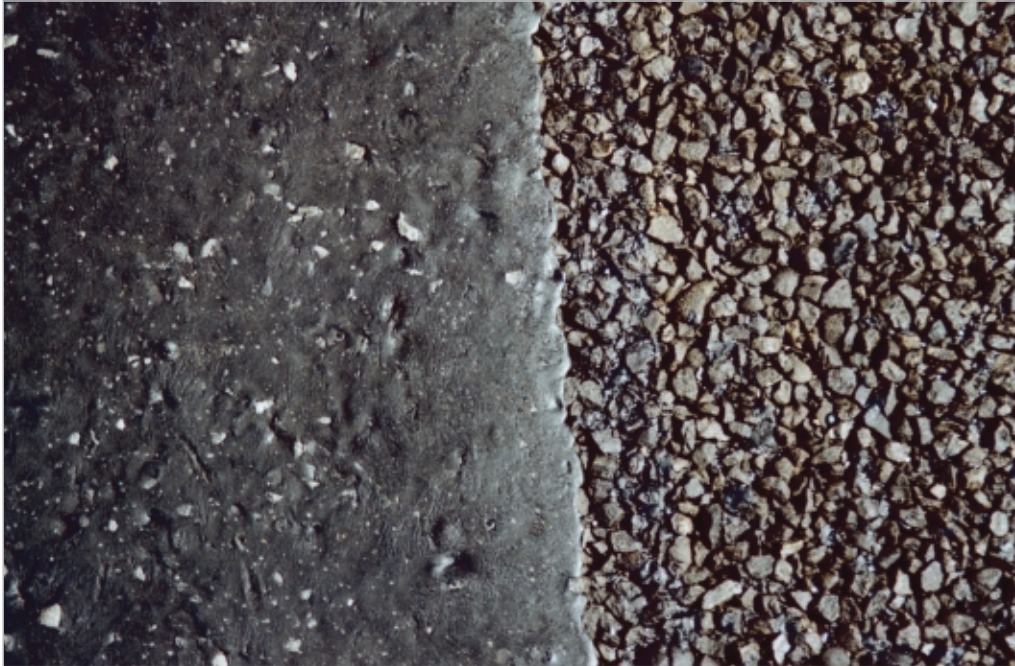
Figure 7-12 A chipseal that is seriously flushed and requires restoration of texture. Left side shows flushing several millimetres thick above the original chip surface, exacerbated by many layers of grit that have been applied to mop up bleeding binder. Right side shows the same seal after water blasting. The original surface with adequate texture depth has been restored.
