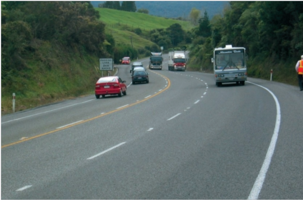
Figure 6-6 A chipseal on climbing lanes where high speed traffic passes heavy vehicles.
