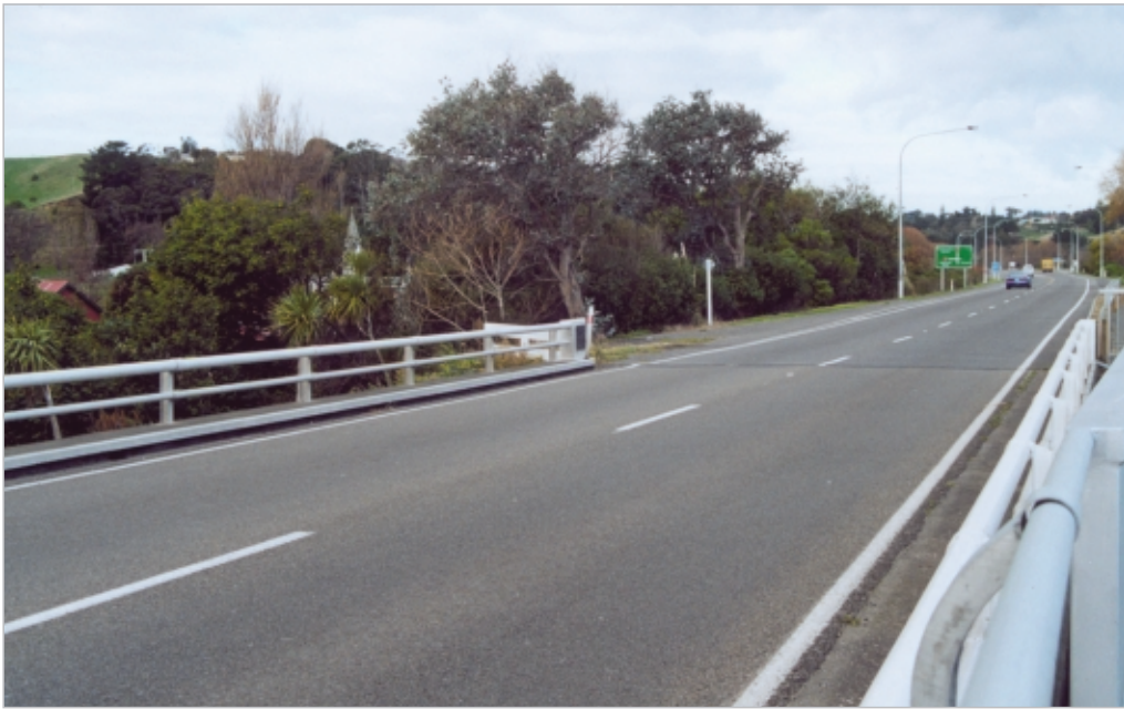
Figure 6-8 An approach road that is consistent with the bridge deck surfacing.
