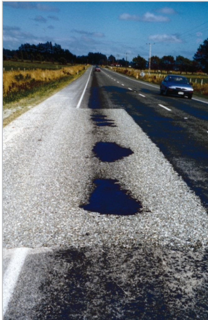
Figure 4-18 A flushed and tracked repair patch.
