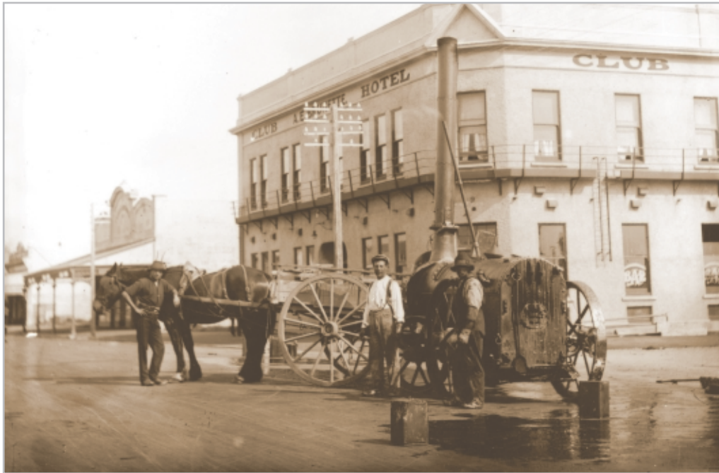
Figure I-4 Draughthorse-drawn bitumen hand sprayer ready for sealing the main street of Opunake, Taranaki, in the 1920s. Photo courtesy of Feaver Collection, Puke Ariki Museum Archives, New Plymouth
