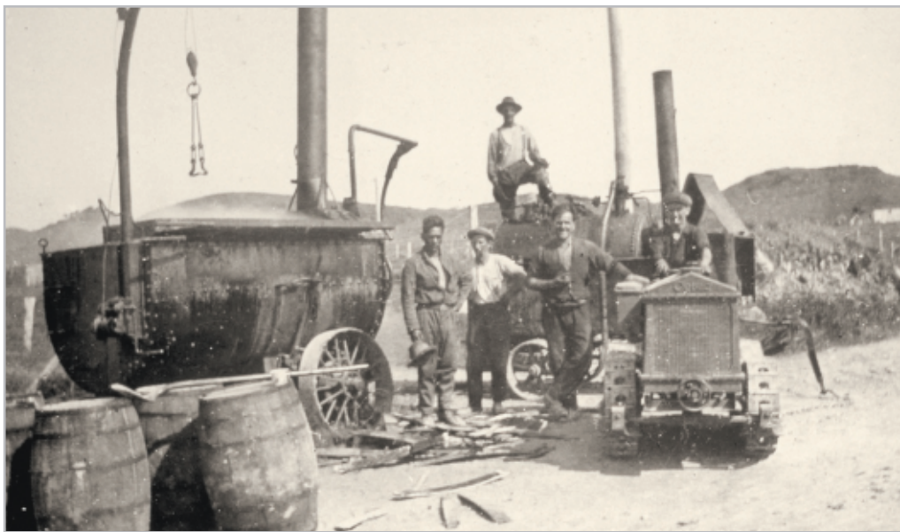
Figure 1-3 This bitumen heating kettle (left) being used in Taranaki was the way to heat bitumen in the 1920s. The fire, stoked with staves from empty bitumen barrels, was in the firebox under the kettle. The firebox gases passed around all sides of the kettle. Photo courtesy of John Matthews, Technix Group Ltd
