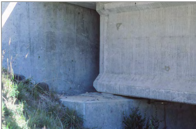
Figure C5B.3: Abutment seating showing sliding bearings (note lack of transverse restraint)
