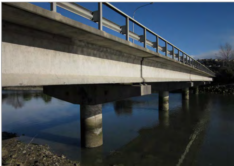
Figure C5A.1: Maitai River Bridge (looking south)
