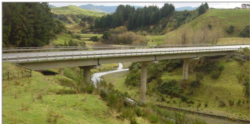
Figure C5B.1: Mangatewai-iti River Bridge looking to north
