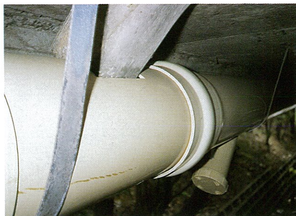
Figure 7.8: Replacement system with inspection and jetting point.
