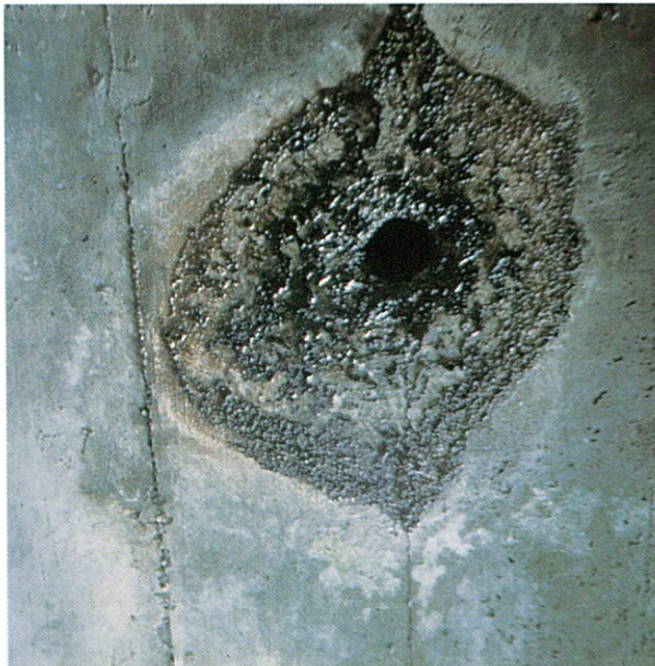
Figure 7.3: Drainage outlet discharging water onto concrete deck soffit.
