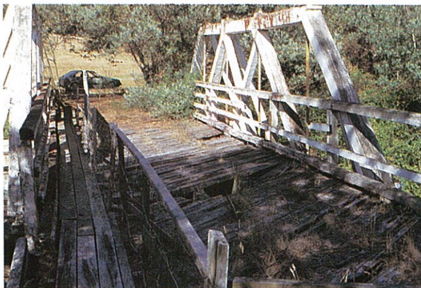
Figure 5.18: Old truss bridge beyond its life limit for vehicles. Some old bridges have a heritage value and deserve preservation, possibly for pedestrian use.
