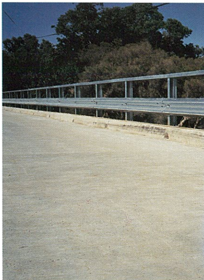
Figure 5.26: Concrete overlay complete.
