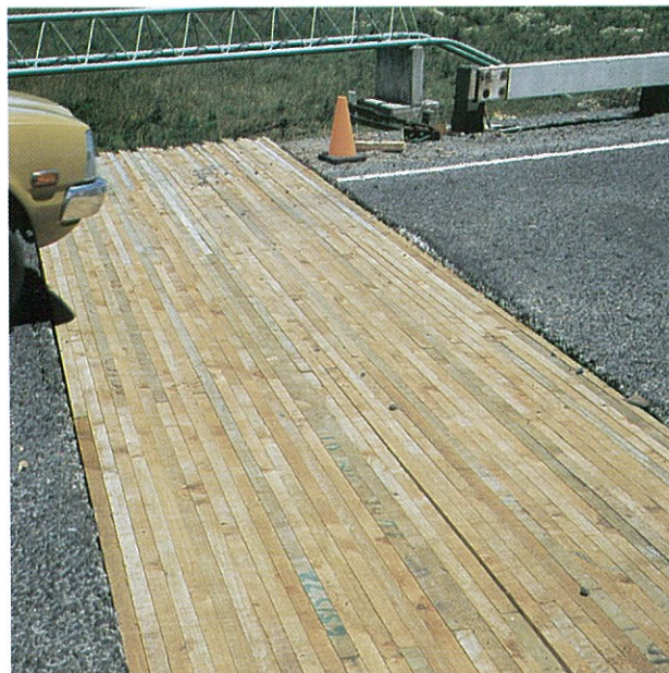
Figure 5.19: Replacement sections of radiata pine nail-laminated deck.
