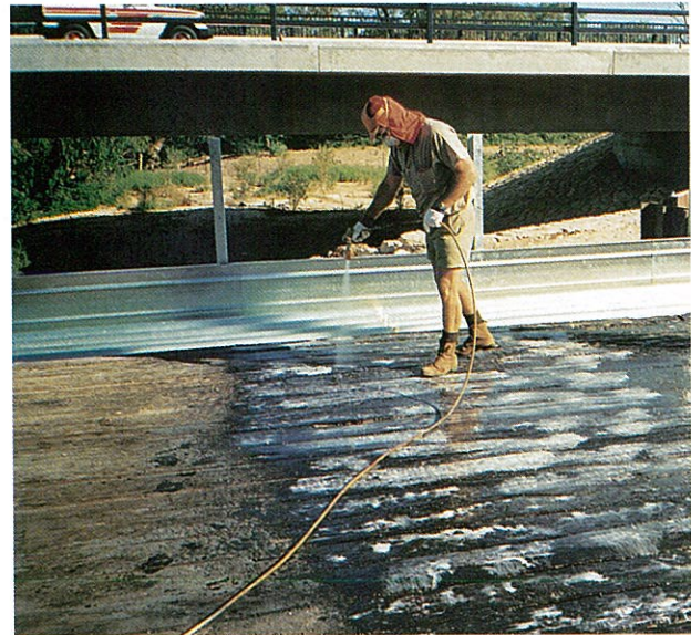
Figure 5.24: Application of diffusible fungicide (Boracol) prior to installing concrete overlay.
