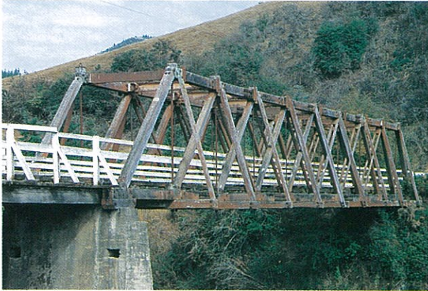
Figure 5.1: Timber truss bridge comprises timber members bolted together.
