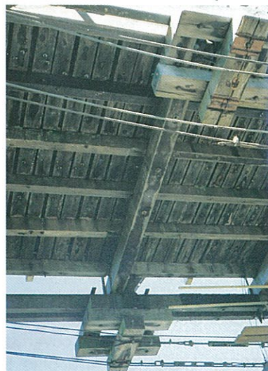
Figure 5.23: Reinforcement of truss with tensioned wire rope.
