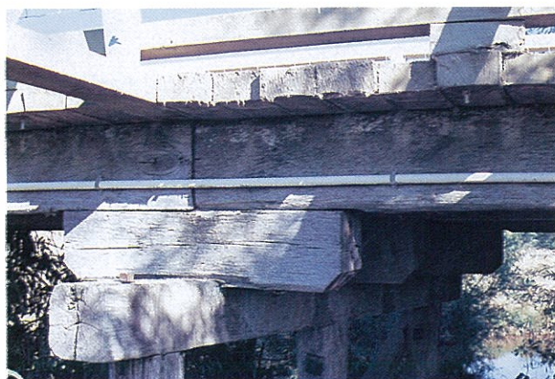
Figure 5.16: Old timber bridge with relatively new treated radiata pine decking.
