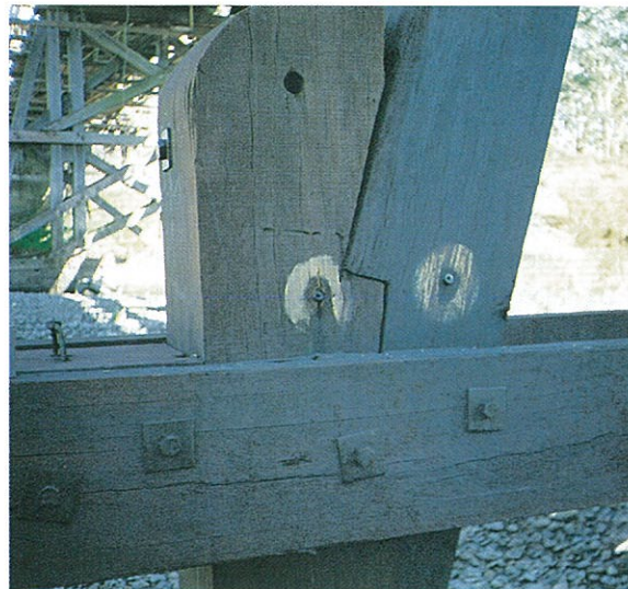
Figure 5.21: Repair to base of raking pier member.
