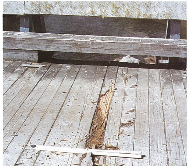
Figure 5.7: Decay in laminated macrocarpa deck after 10 years.
