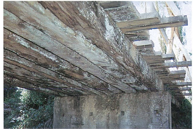
Figure 5.12: Old timber superstructure with an assemblage of beams.
