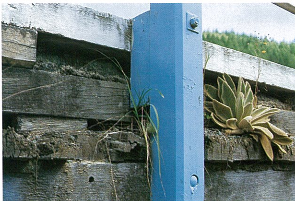
Figure 5.9: Drill hole, accumulation of road gravel, vegetation growth, and decay in deck planks.
