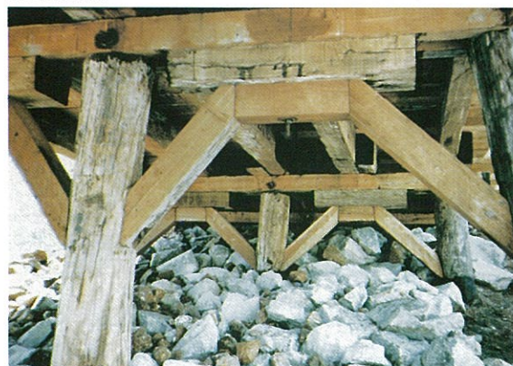
Figure 5.22: New bracing provides additional support to an old hardwood superstructure.
