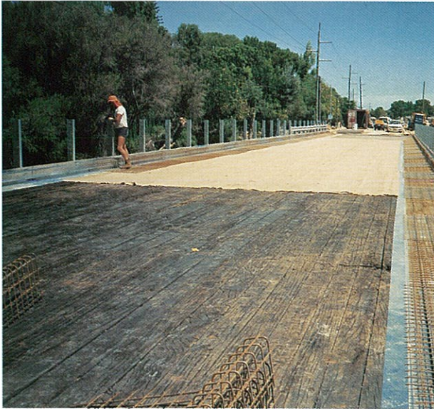
Figure 5.25: Preparation for concrete overlay.
