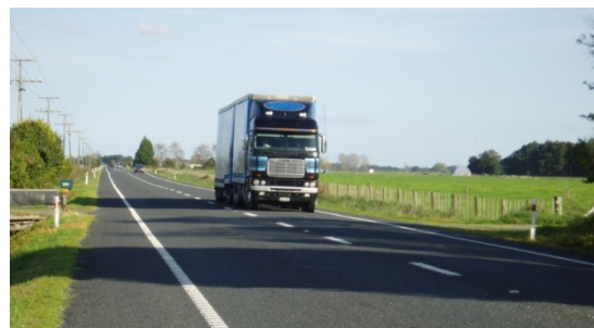
Figure 4. Sufficient shoulder width is needed to accommodate cyclists where ATP roadmarkings are used
