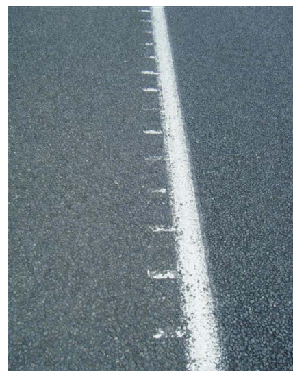
Figure 7. ATP rib removal via grader blade
