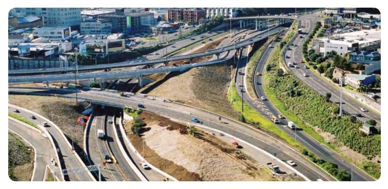
Construction of the multi-million dollar project started in January 2004, comprising the four new links between SH1 and SH16, two new off-ramps to Nelson Street from the Southern and Northwestern Motorways, and new lane layouts to make the motorway safer and more intuitive to use.
