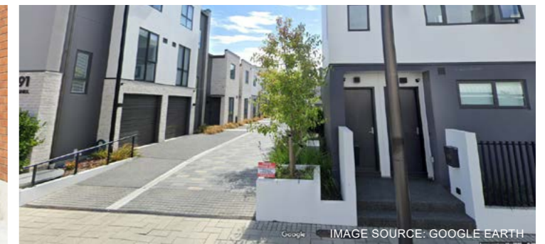
IMAGE SOURCE: GOOGLE EARTH 191 CASHEL STREET, CHRISTCHURCH
