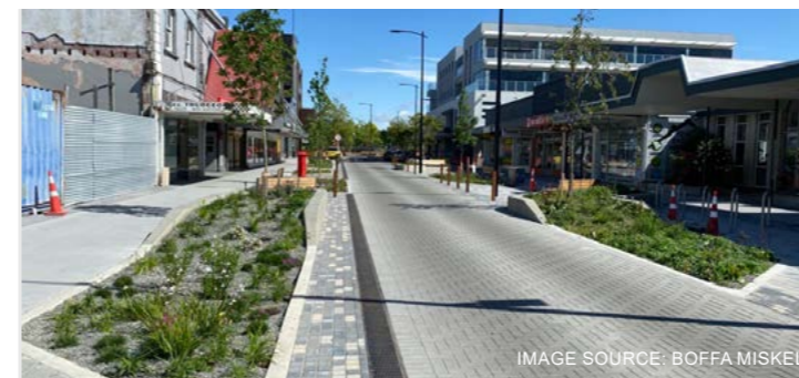
IMAGE SOURCE: BOFFA MISKELL TANCRED STREET, ASHBURTON
