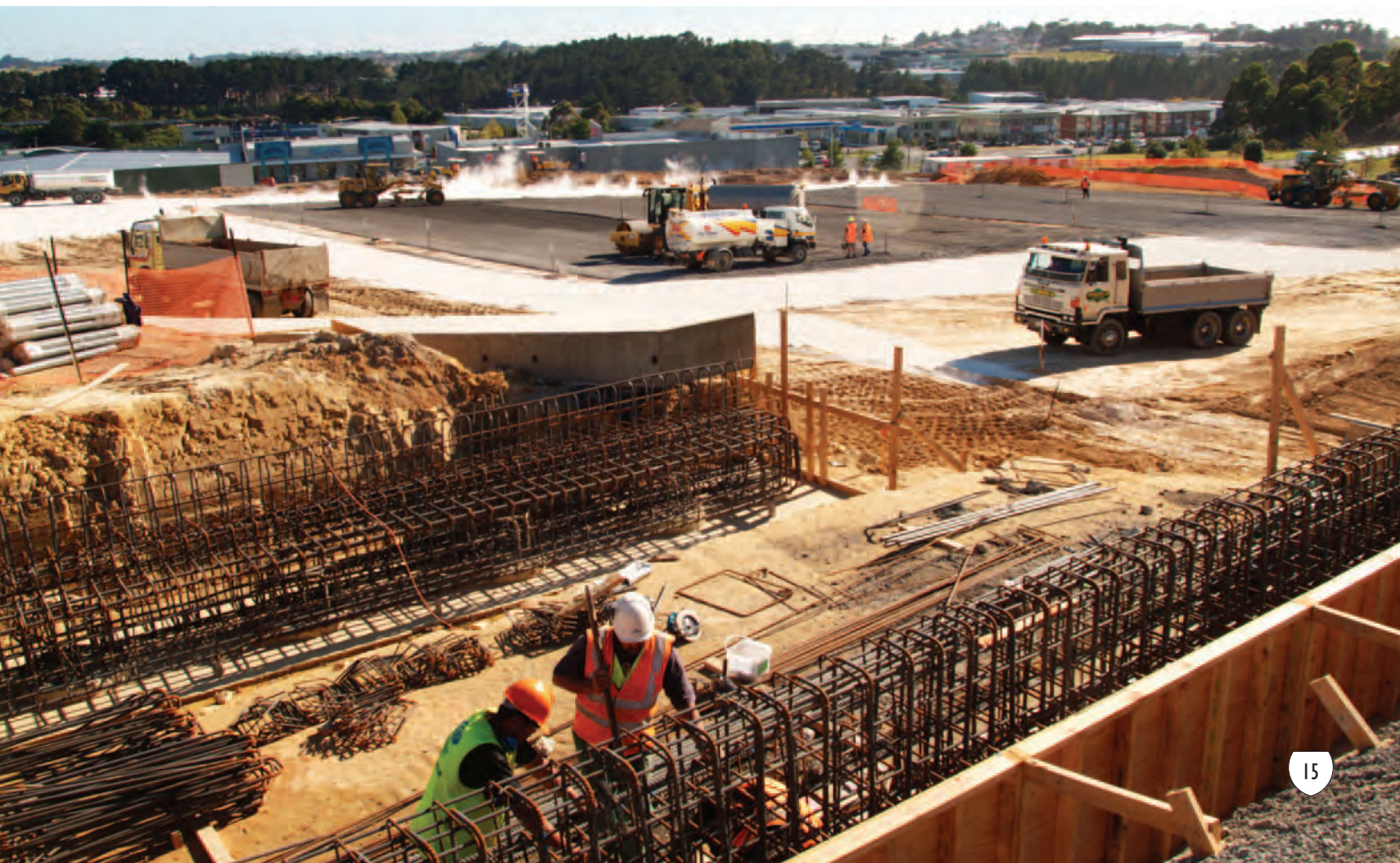
Construction progress on the SH1 Northern Busway project.
