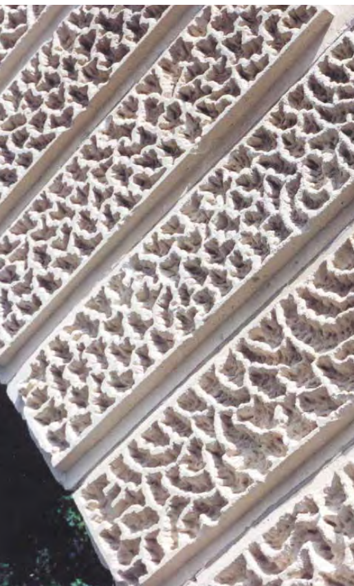
Detail of Waianakarua Bridge SH1
