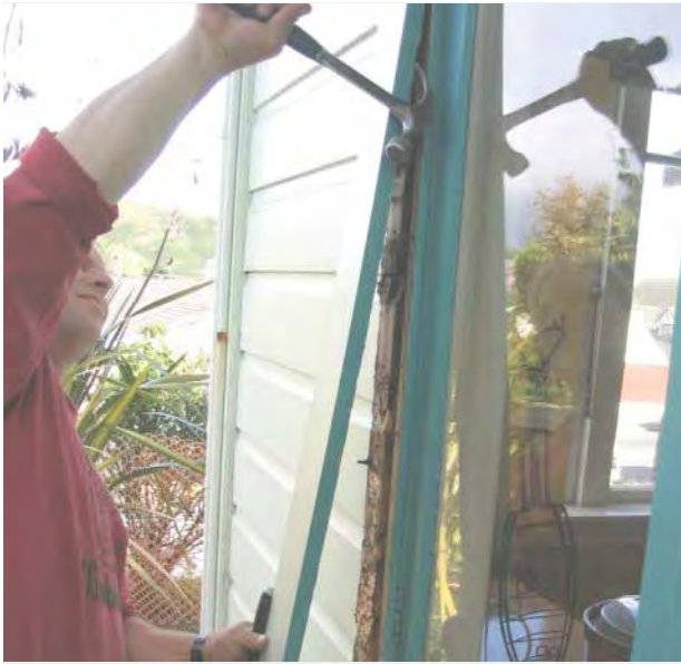
Fitting special glass to a Paremata house to reduce traffic noise from the widened highway.
