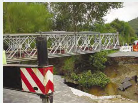
Below: The Bailey bridge makes the connection.
