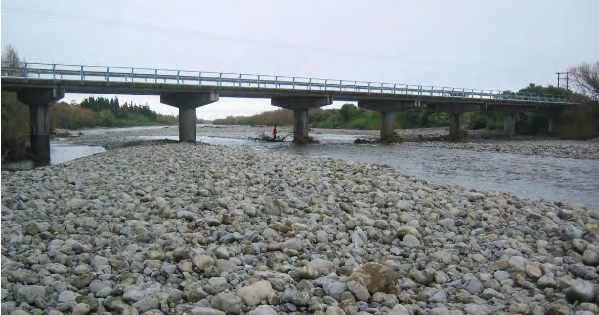
Figure 4.1 SH 2 Tauherenikau River Bridge
