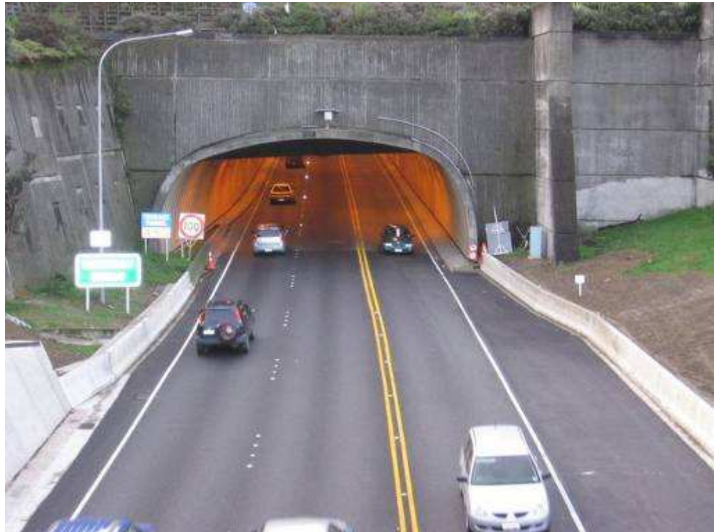
Figure 4.3: The southern portal of the Terrace tunnel (looking north).
