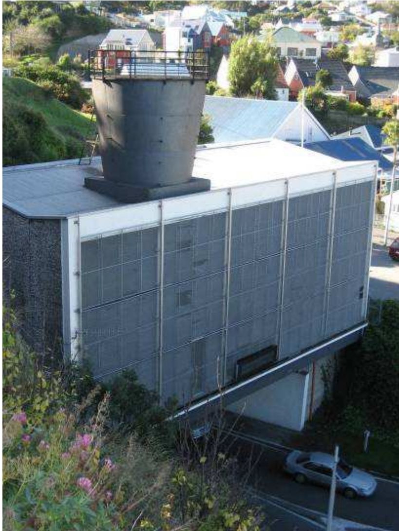
Figure 5.6: View of the southern portal of the Lyttelton tunnel showing the stack, looking north-east. The homes in the middle distance are approximately 100 m away.
