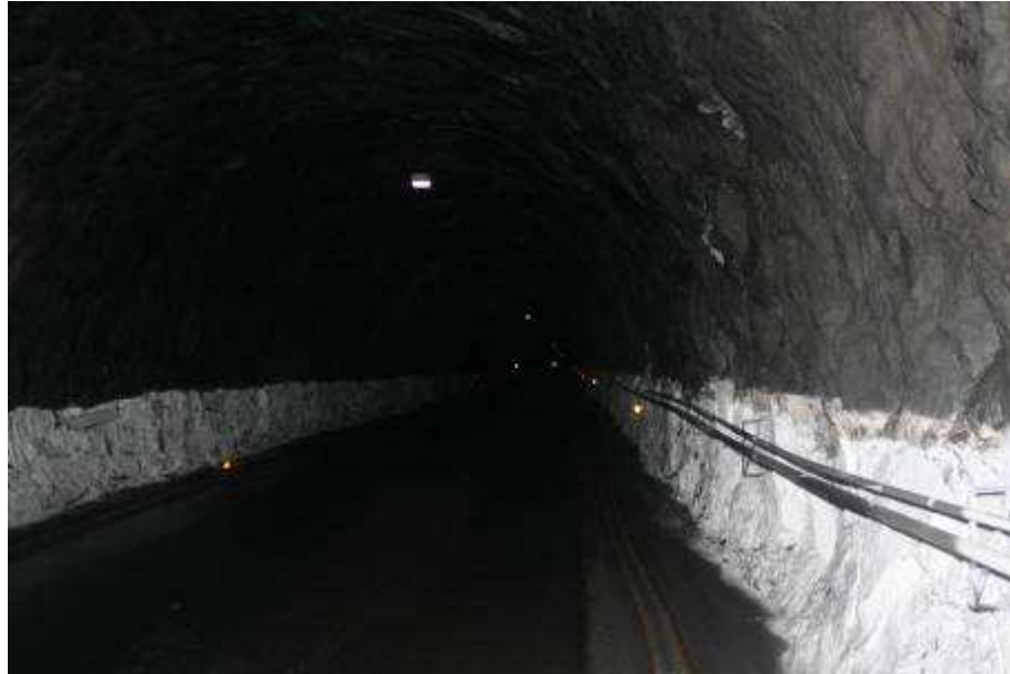
Figure 6.5: Homer tunnel interior view.
