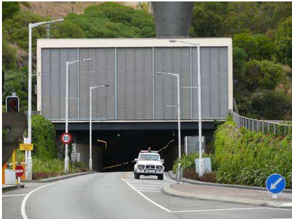
Figure 5.3: Christchurch end of the Lyttelton tunnel. The screens stand in front of the intake (left) and exhaust (right) fans, with the exhaust stack visible top right of centre.
