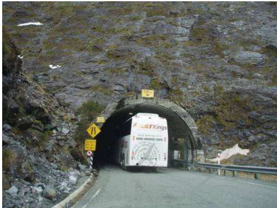
Figure 6.3: Milford Sound (western) end of the Homer tunnel.
