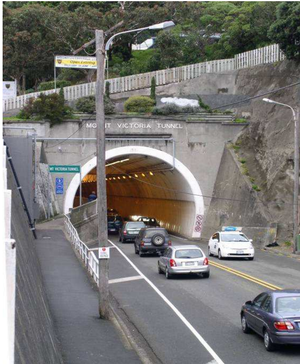
Figure 3.3: Western portal of the Mt Victoria Tunnel showing pedestrian walkway.
