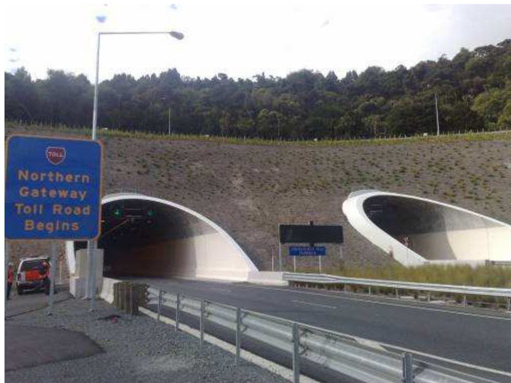
Figure 7.3: View of the Johnstone's Hill twin tunnels from the northern end.
