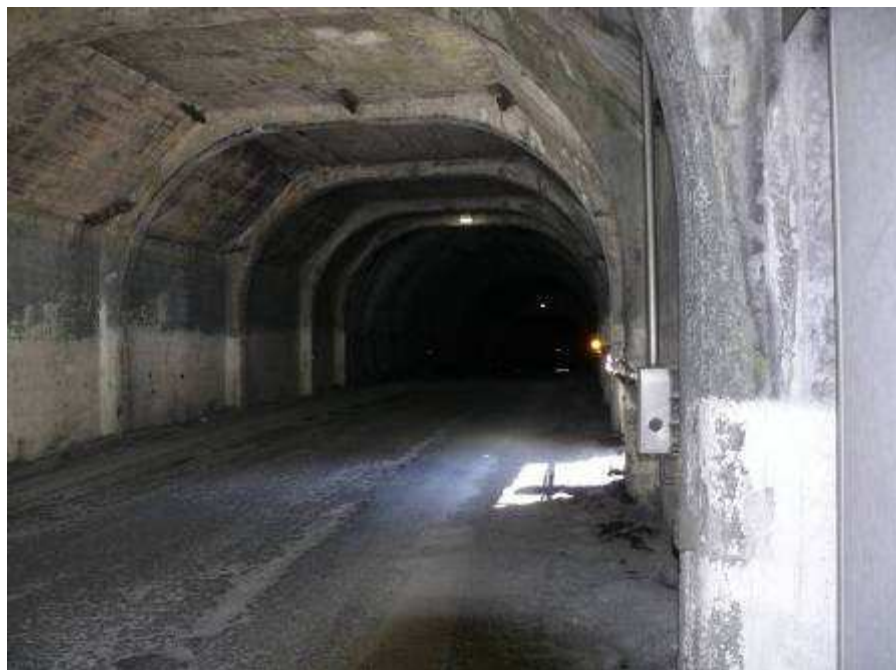
Figure 6.4: Homer tunnel at the Te Anau (eastern) portal.
