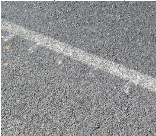
ATP roadmarking of the eastbound edgeline (ATP east)
