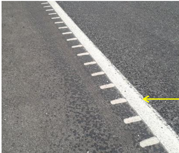
Figure 2.1 Example of in-lane reseal with the edge of the reseal within the normal/flat edgeline
