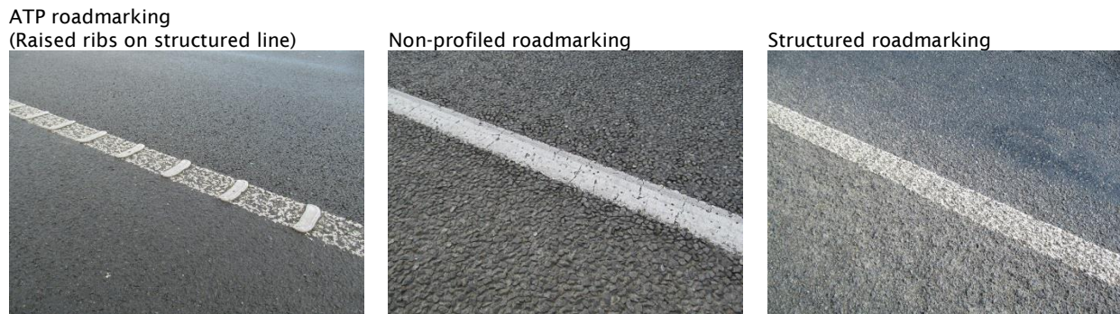
Figure A.2 Samples of the three roadmarking types measured
