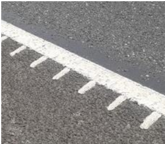
Figure 4.2 ATP roadmarking post-in-lane reseal
