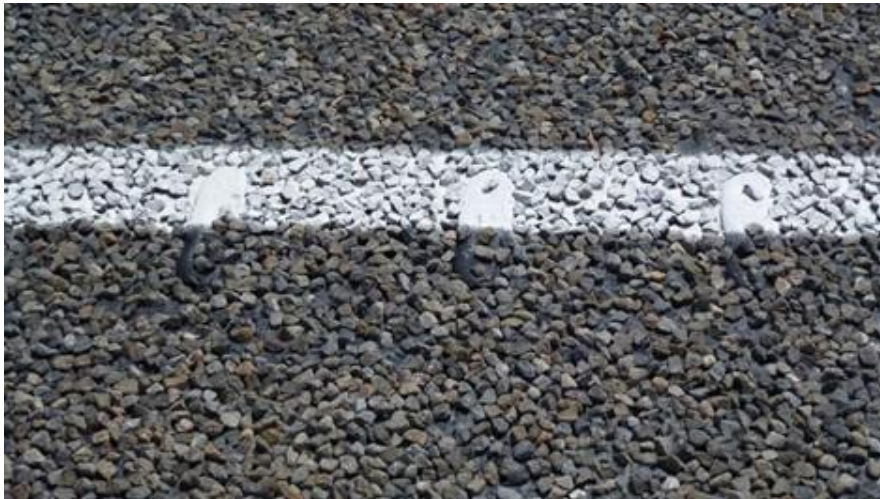
Figure 4.11 (Good condition) ATP roadmarkings post-reseal with grade 3 chip (example 4)
