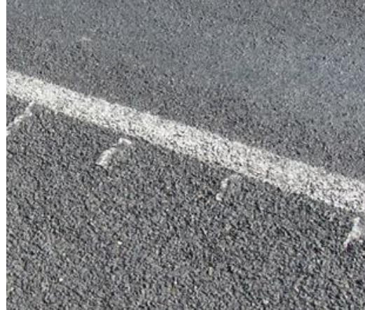
ATP roadmarking of the westbound edgeline (ATP west)
