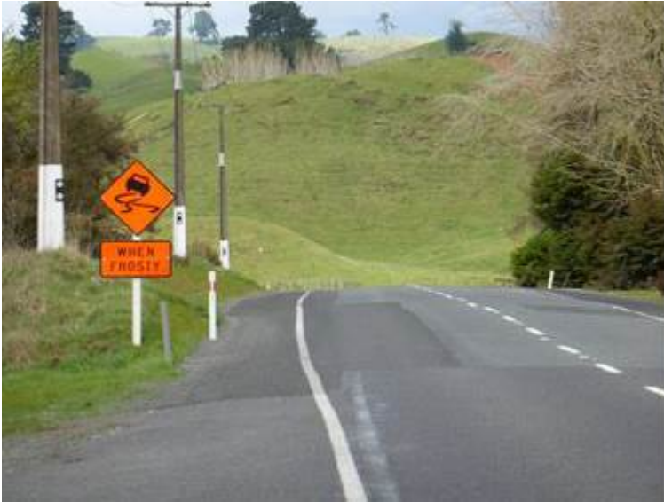
Figure A.3 Grass or soil verges blocking water from flowing away from the pavement are often the main cause of early phase permanent deformation as an example from A83 in Scotland shows
