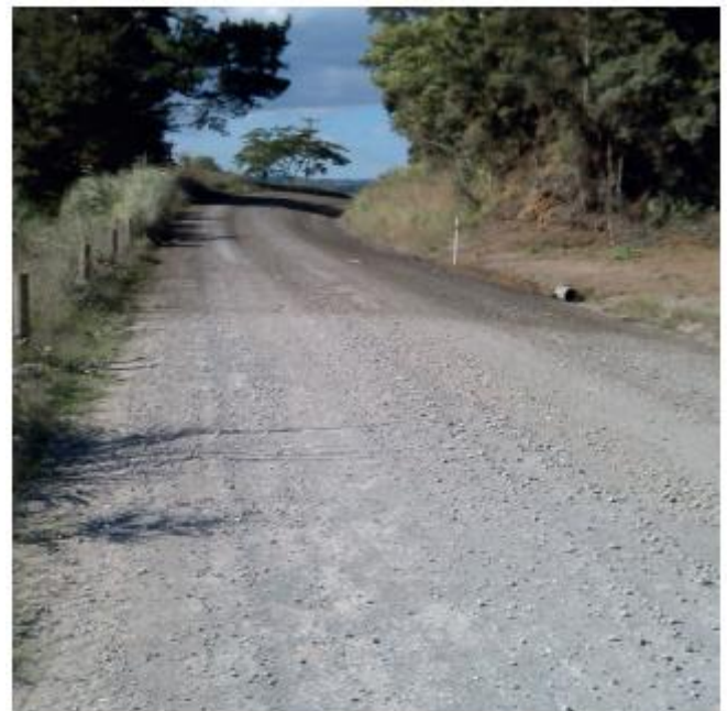
Application of magnesium chloride to Matarau Road
