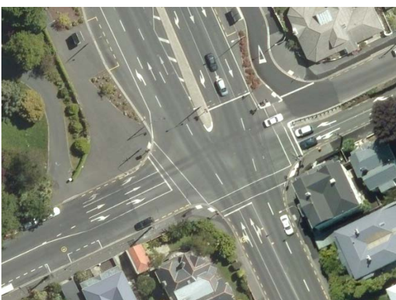
Figure 6.3 Aerial image of Stuart Street, London Street and Arthur Street intersection, Dunedin
