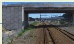
Korokoro Crescent overbridge • 3.5m-wide cycle path • 1.8m high security fence and lighting
