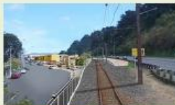
North of Parliament Street rail underpass • 3.5m-wide cycle path • 1.8m-high security fence and lighting • 1.1m-high balustrade to highway • lighting and security cameras integrated with underpass structure
