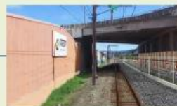
Dowse interchange overbridge • 3.5m-wide cycle path • 1.8m-high security fence and lighting • 1.5m-wide southbound cycle bypass to State Highway 2 • 1.2m-high bypass markers • panels with lighting beneath the overbridge to improve safety
