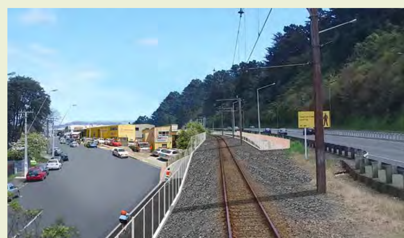
North of Parliament Street rail underpass ▪ 3.5m-wide cycle path ▪ 1.8m-high security fence and lighting ▪ 1.1m-high balustrade to highway ▪ lighting and security cameras integrated with underpass structure
