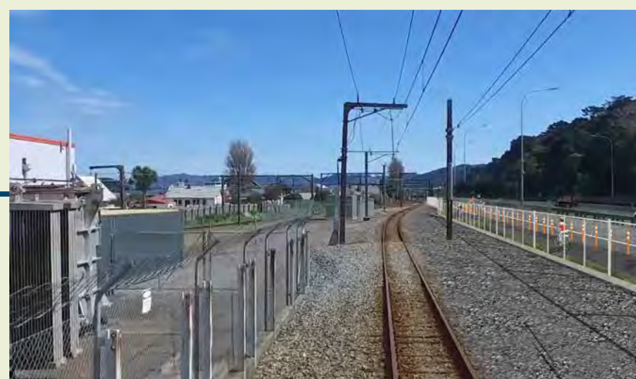
Dowse interchange bypass - south connection ▪ 3.5m-wide cycle path ▪ 1.8m-high security fence and lighting ▪ 1.5m-wide southbound cycle bypass
