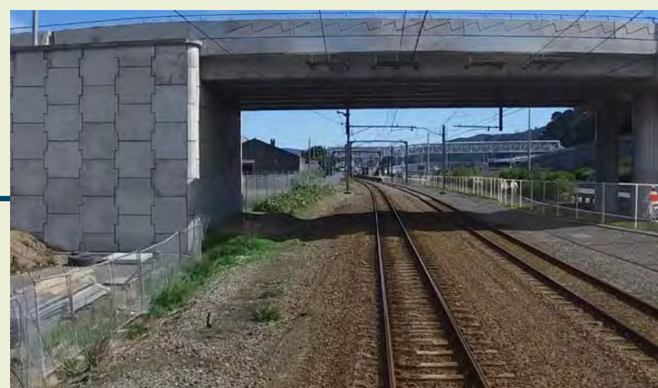
Korokoro Crescent overbridge ▪ 3.5m-wide cycle path ▪ 1.8m high security fence and lighting
