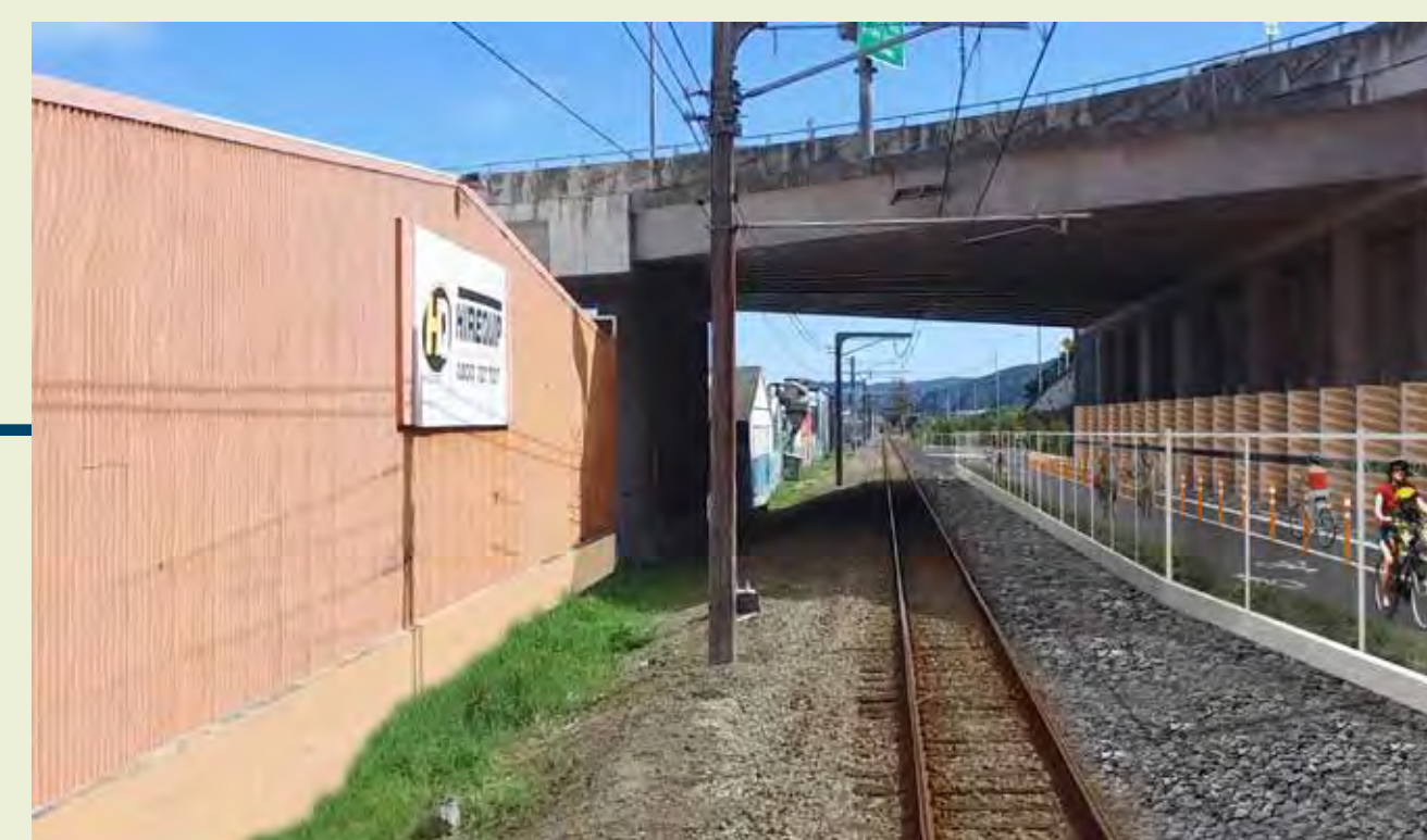
Dowse interchange overbridge ▪ 3.5m-wide cycle path ▪ 1.8m-high security fence and lighting ▪ 1.5m-wide southbound cycle bypass to State Highway 2 ▪ 1.2m-high bypass markers ▪ panels with lighting beneath the overbridge to improve safety
