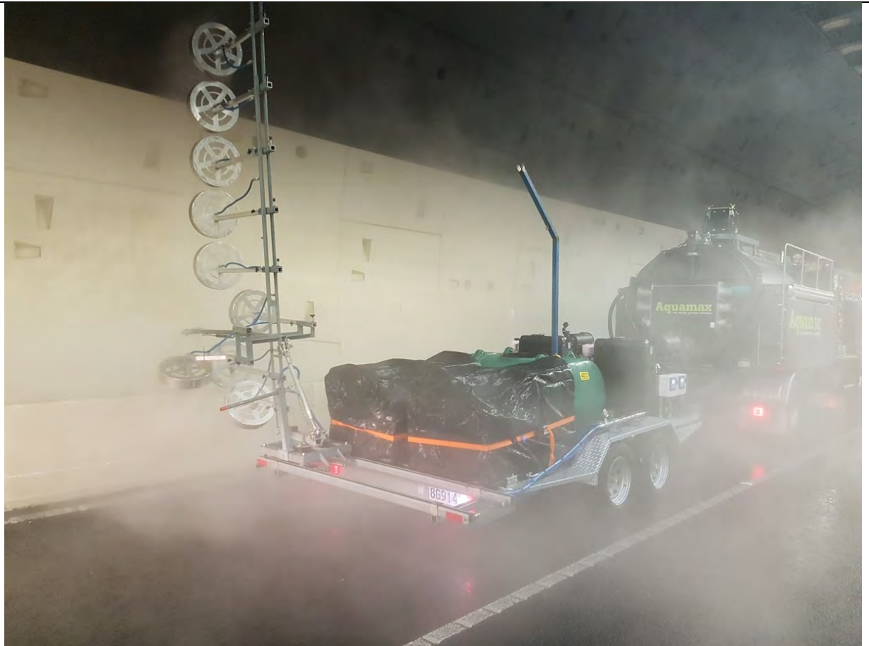
Typical Tunnel Washing Setup
