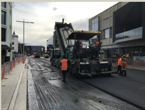
Examples of pavement being laid.
