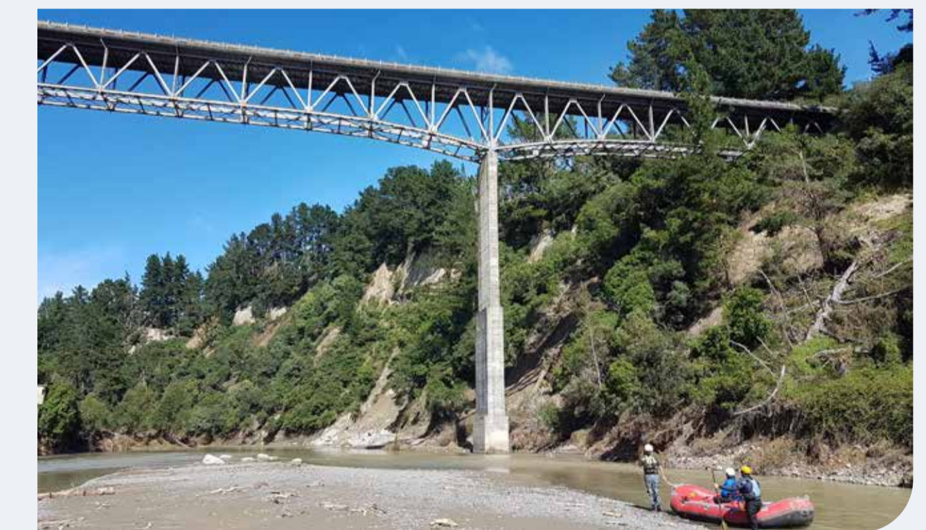
SH5 Mohaka Bridge
