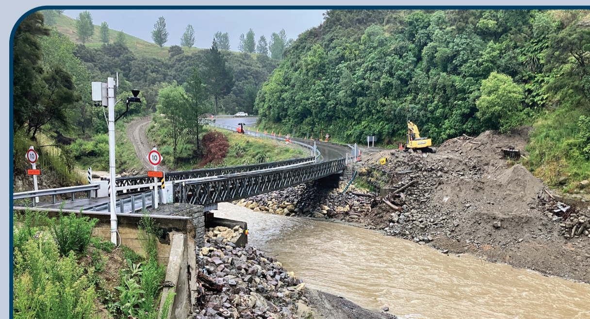
February | The old bridge is demolished
