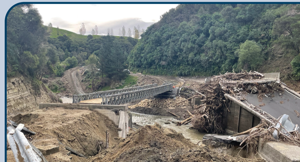
May | A temporary Bailey bridge opened, reconnecting Wairoa and Napier
