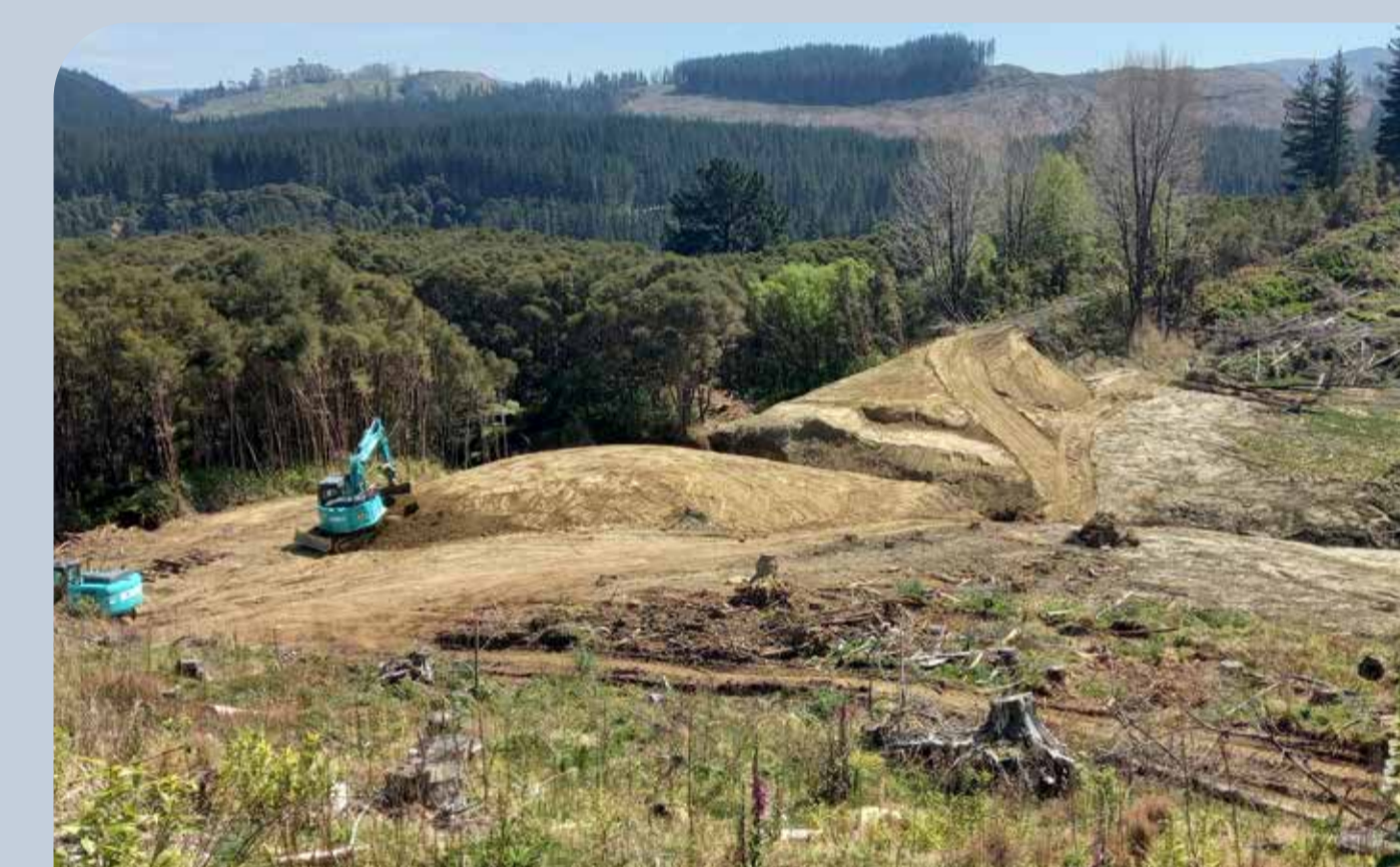
Make Safe works at embankment / culvert failure
