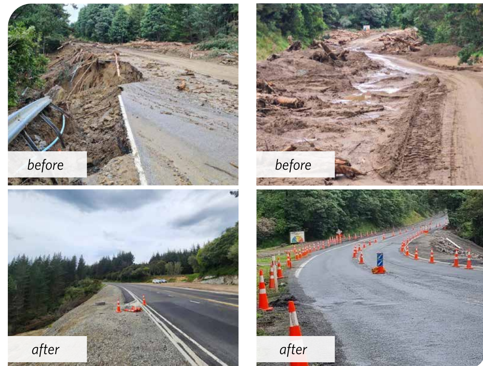
Recovery work in action at SH5 Elands and Esk underslips
