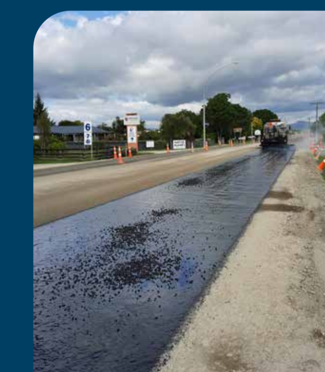
Maintenance work going well
