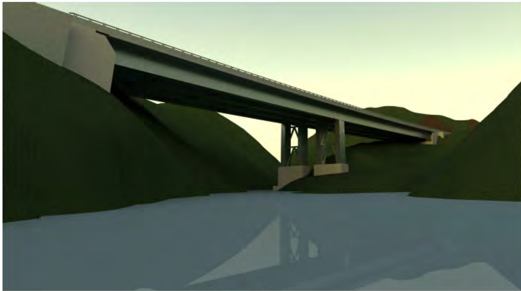
BRIDGE 19 LOOKING SOUTH
