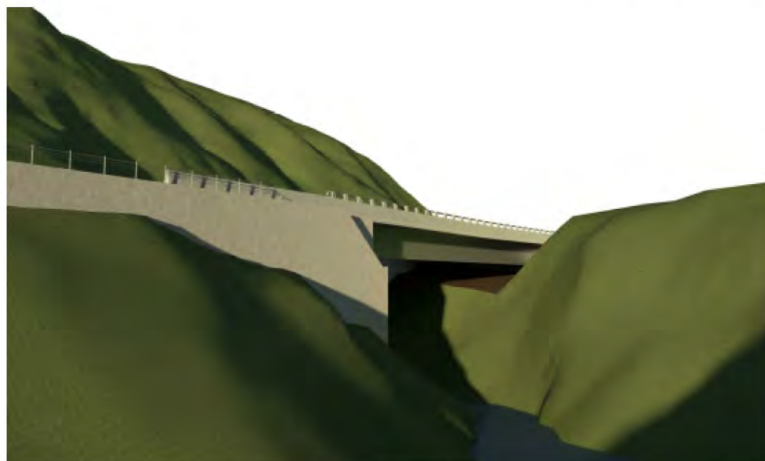
BRIDGE 03 LOOKING NORTH
