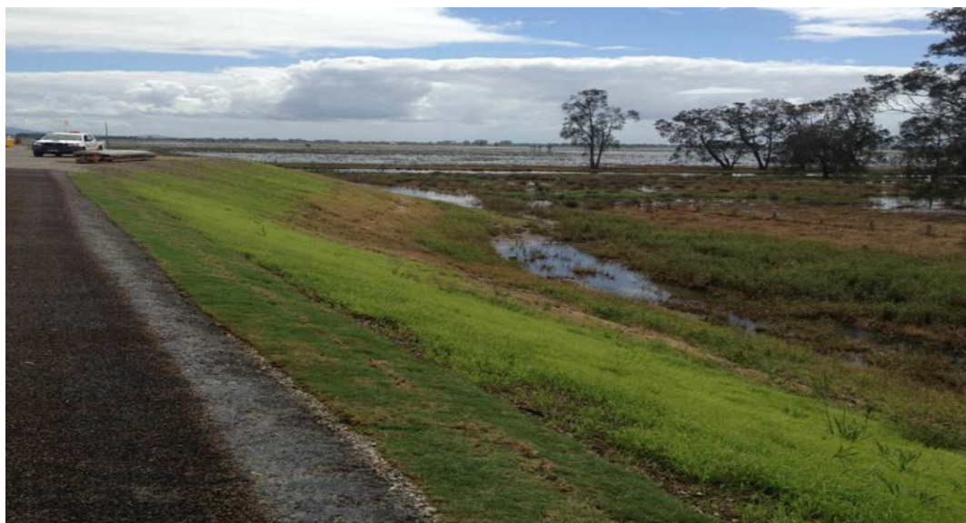
Figure 5 - Recently constructed vegetated batter in sensitive environment
