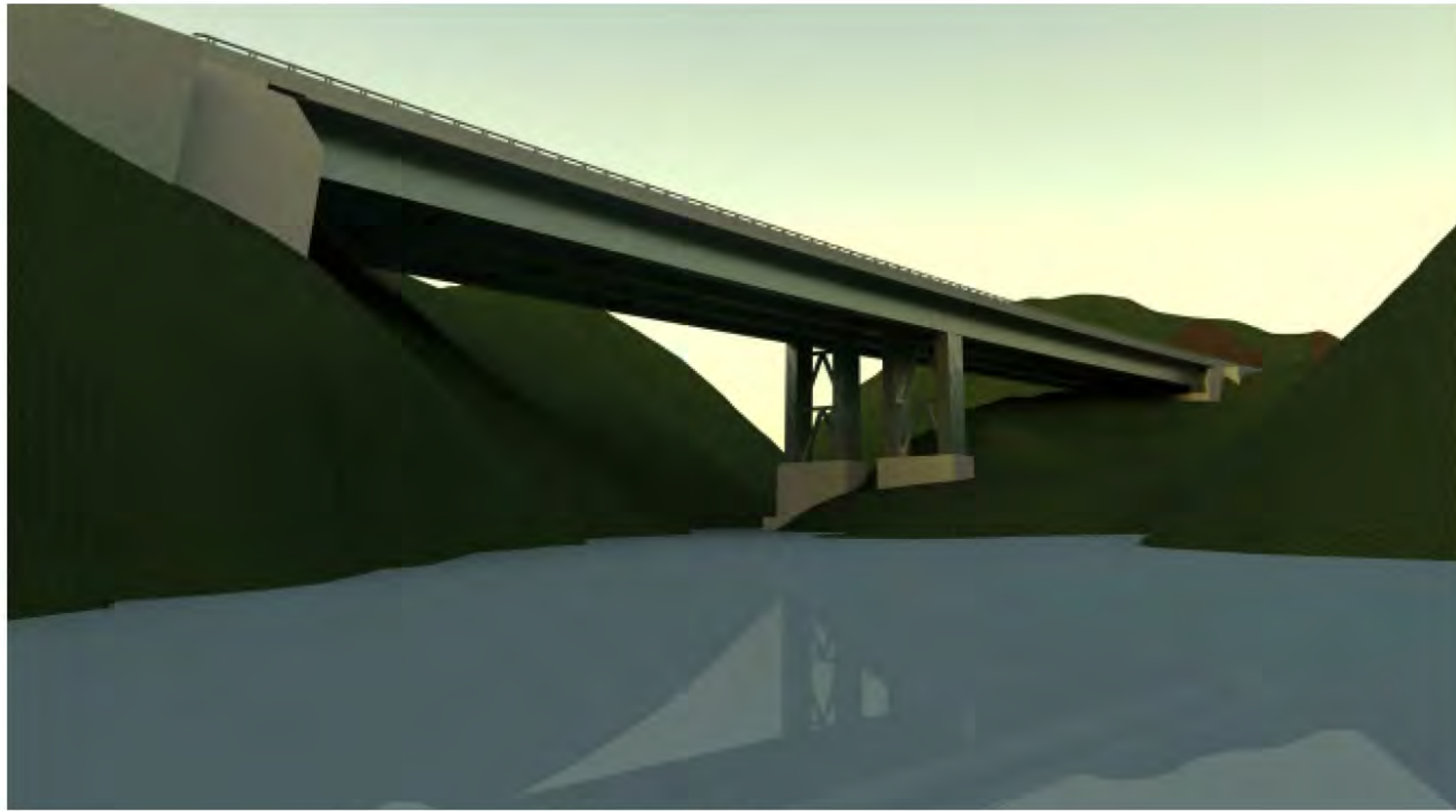
BRIDGE 19 LOOKING SOUTH
