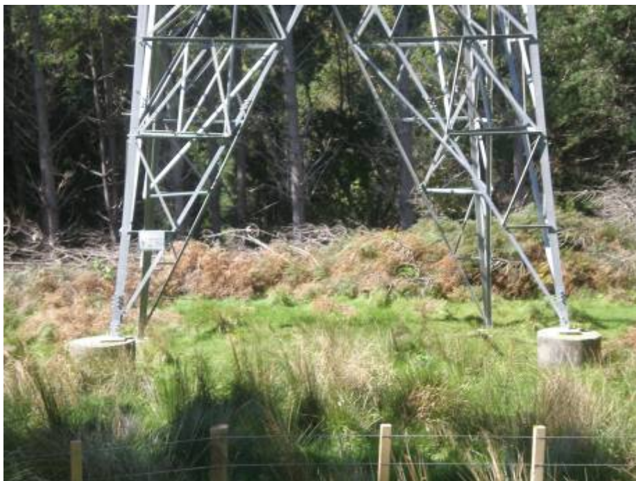
Figure 3.7: Example of Pile Foundations
