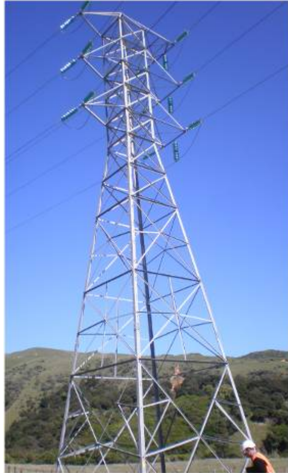
Figure 3.4: Example of a Strain Tower (PKK-TKR A transmission line).
