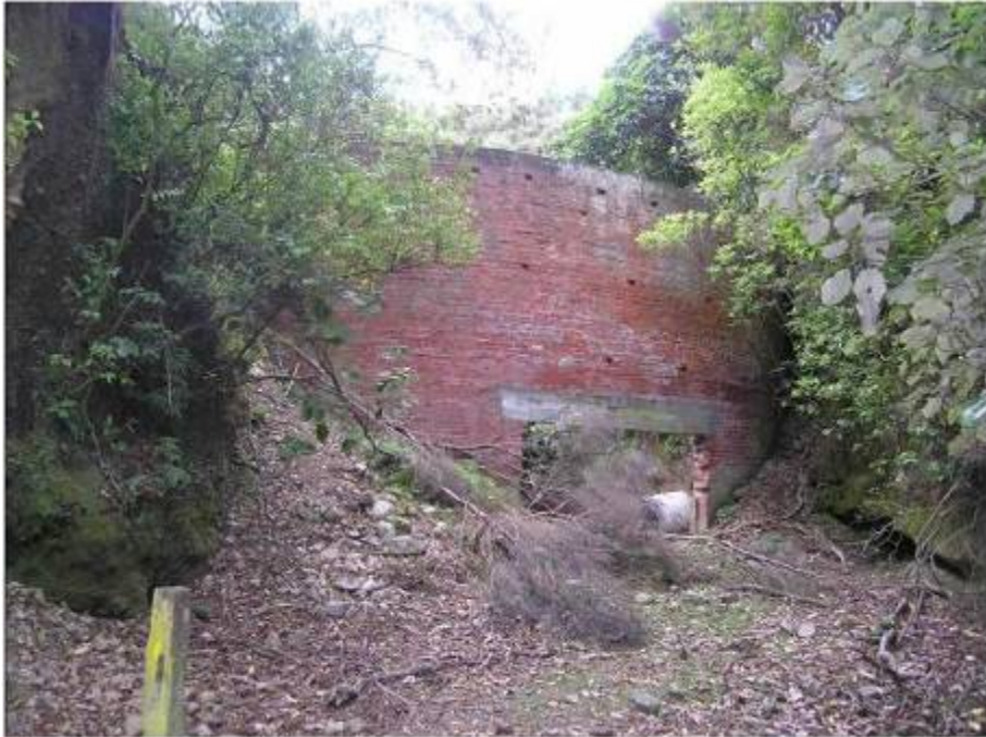
Figure 2.4: Photograph of the Brick Fuel Storage Tank
