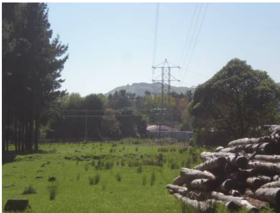
Figure 2.3: Looking Towards Tower 1 and SH1
