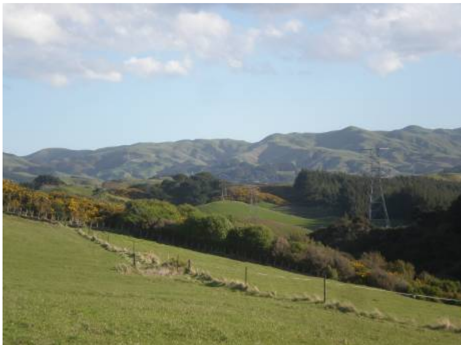
Figure 2.13: View of Towers 38 to 41 from near tower 41 (facing north)
