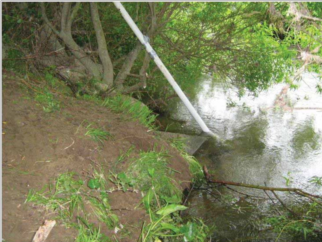
Photo 9-16 Lower reach were logger was installed.
