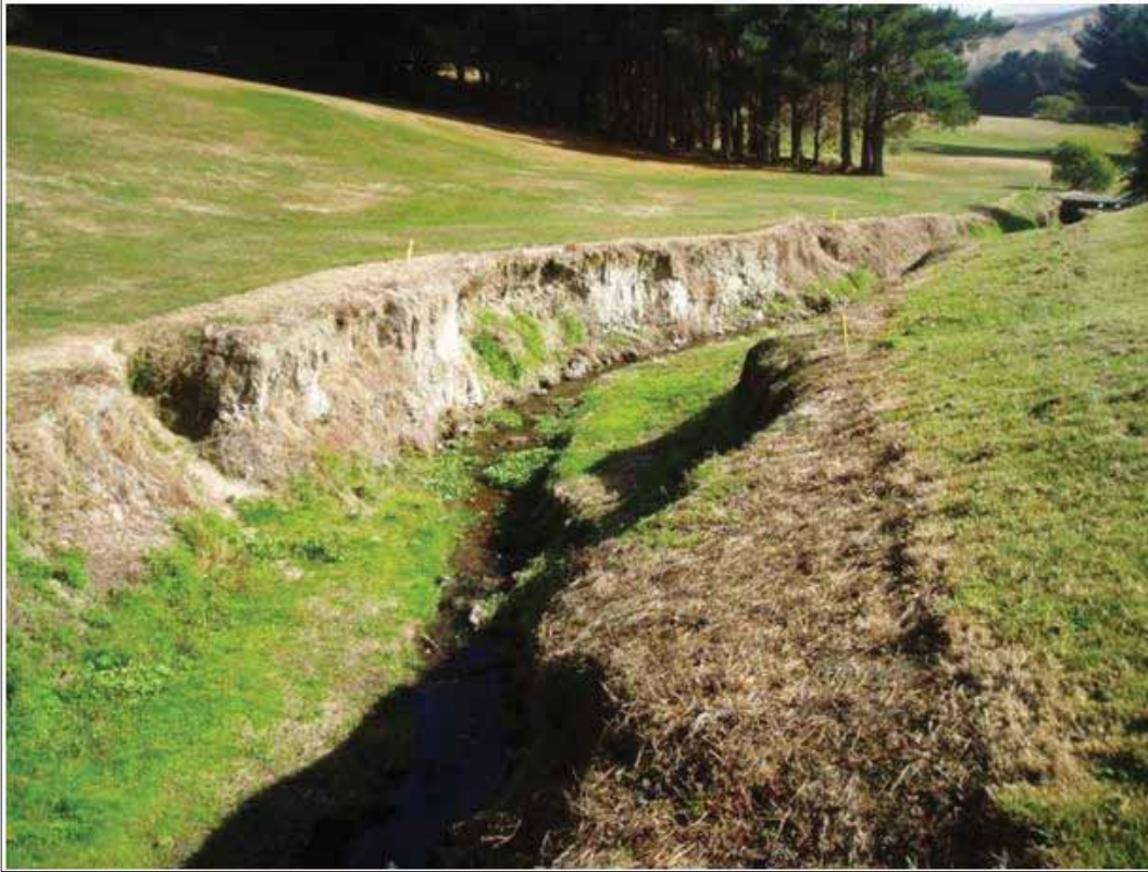
Photo 9-12 A middle reach view through the golf course of the ration. Note the deep set bur small flow and highly managed and modified riparian condition.
