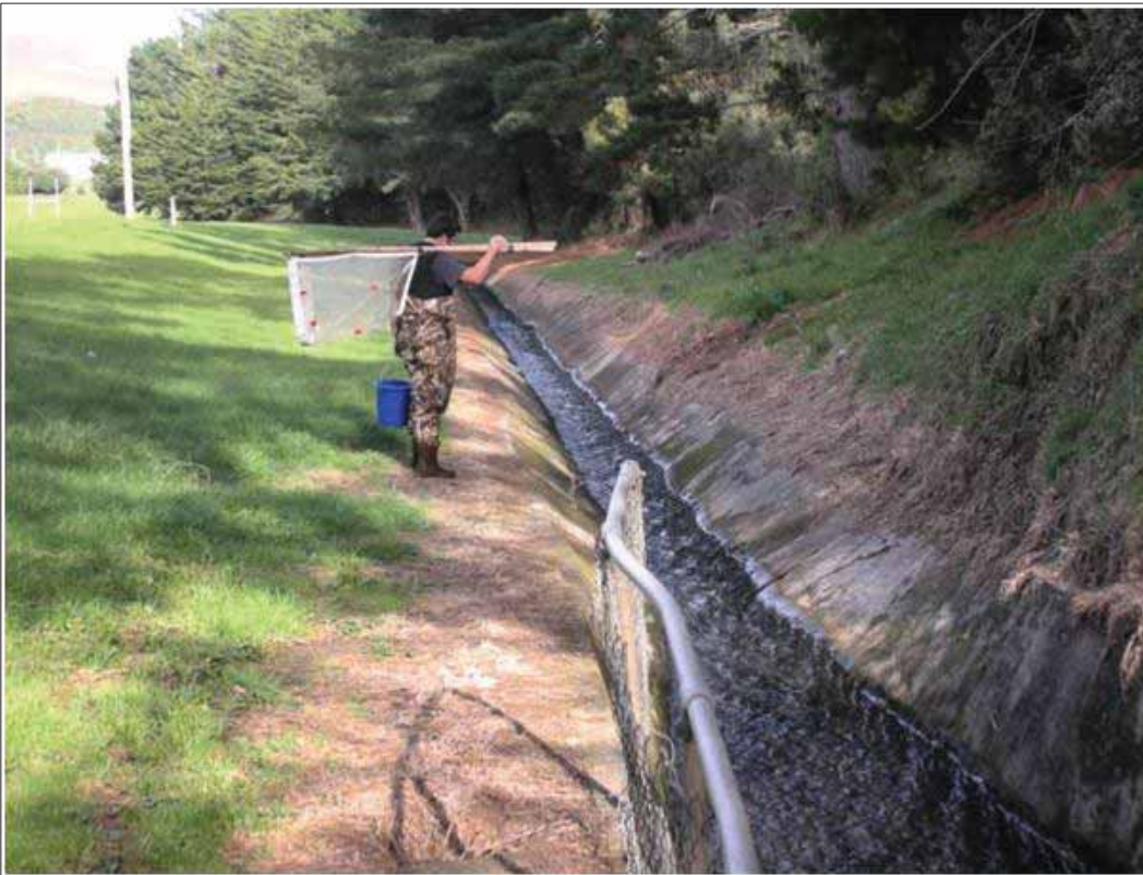
Photo 9-24 Lower Cannons Creek (below ponds) Note a concrete lined "drain"
