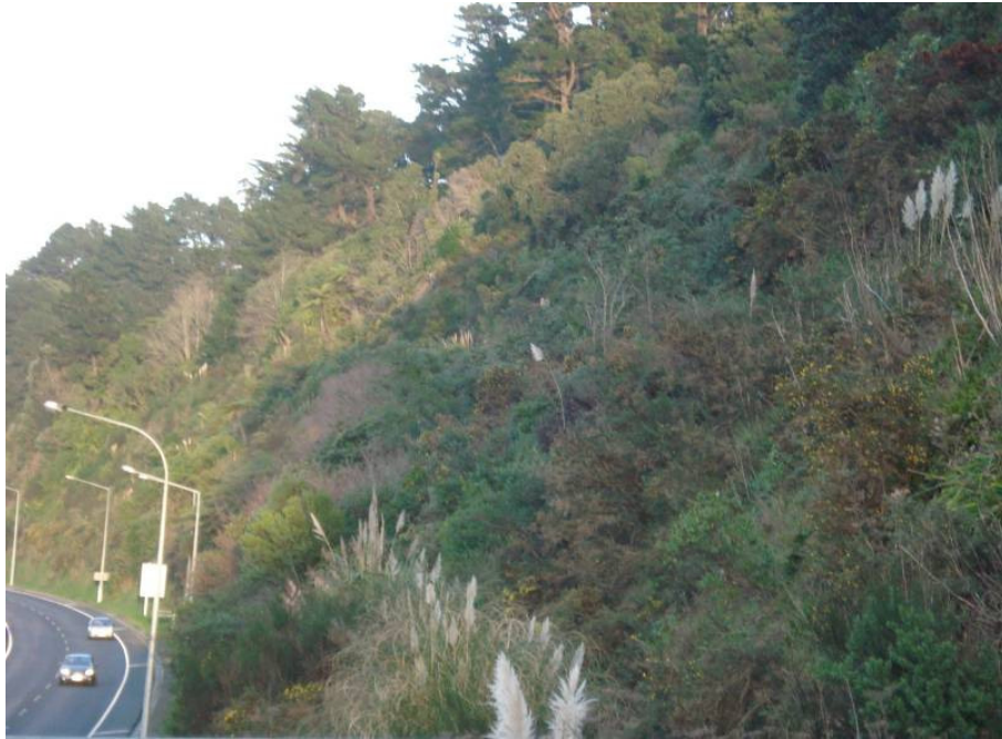
Illustration 3.27 - Rock Cutting with Benches along State Highway 2, after 50 Years
