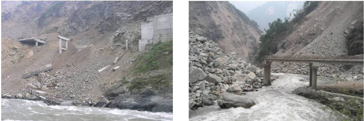
Illustration 3.9 - Viaduct / bridges in steep terrain destroyed by landslides in the Wenchuan Earthquake
