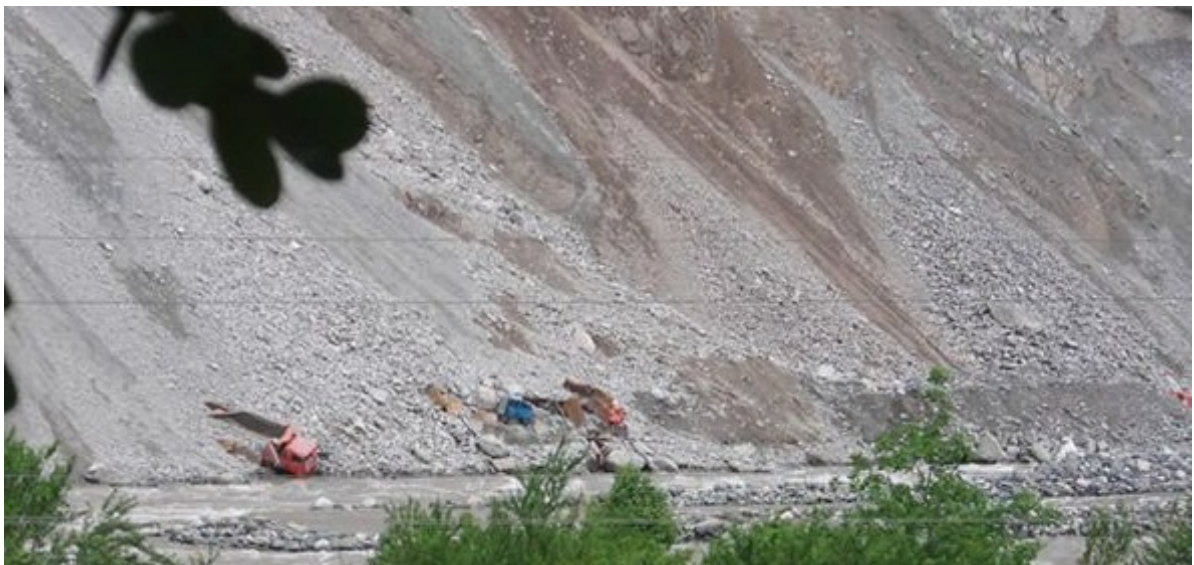
Illustration 3.8 - Highway destroyed by landslides in the 2008 Wenchuan Earthquake, China
