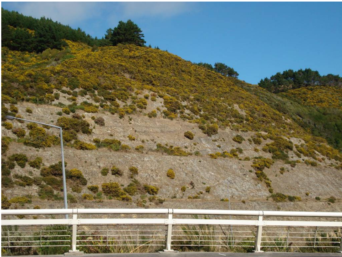
Illustration 3.19 - Benched Cut Slope in Wellington Greywacke at SH 1 Newlands Interchange
