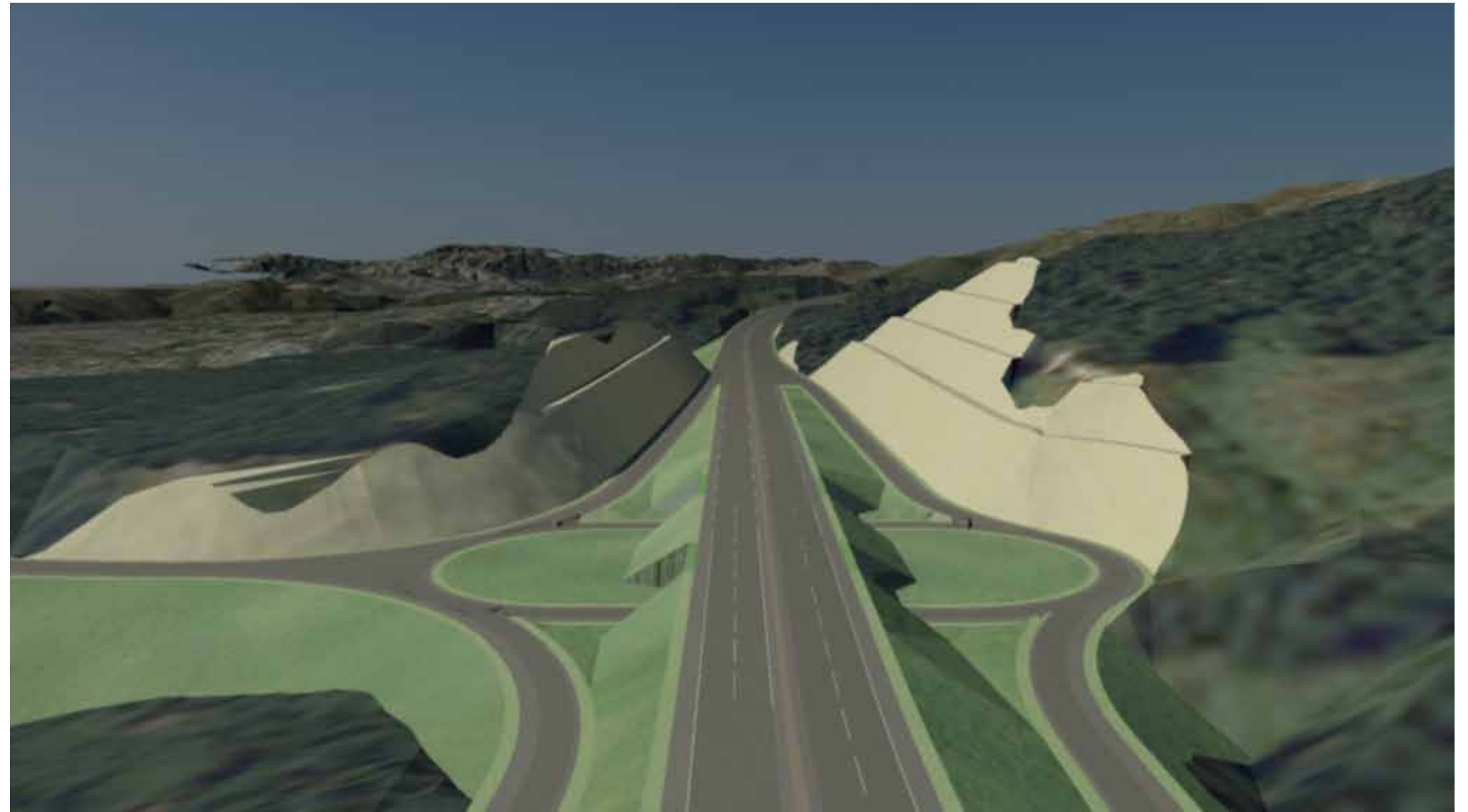
Figure 5.70: Section 9 Kenepuru Interchange Earthworks - View to North-east
