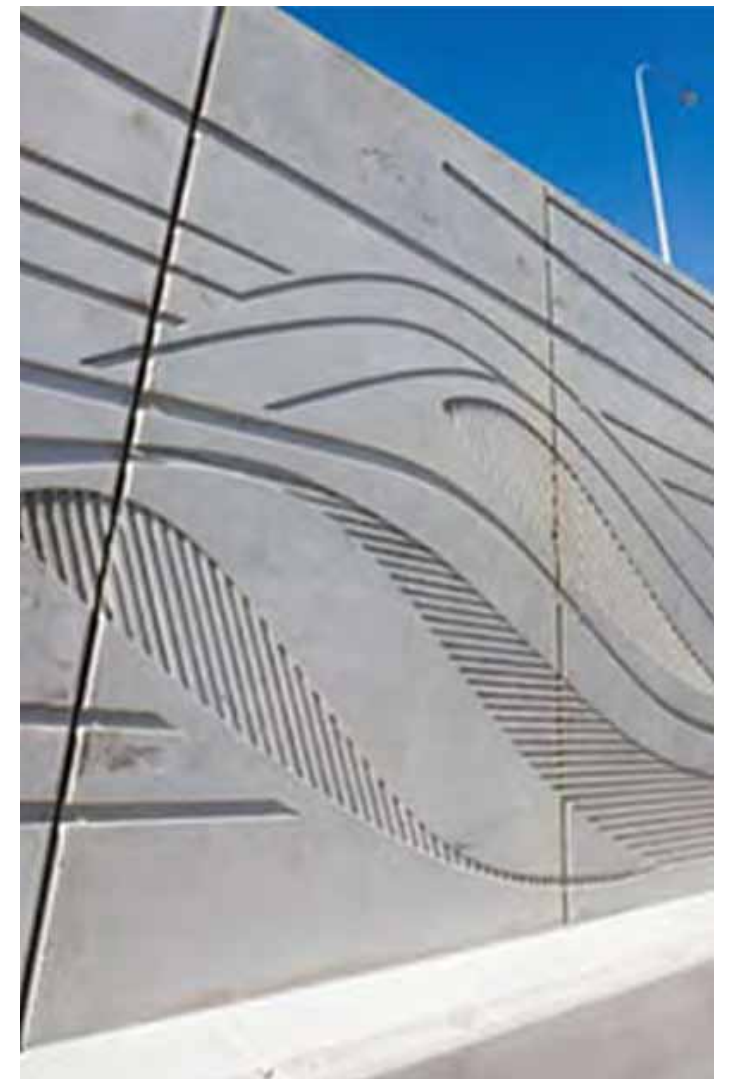
Photo 5.31: Concrete noise wall combined with side barrier
