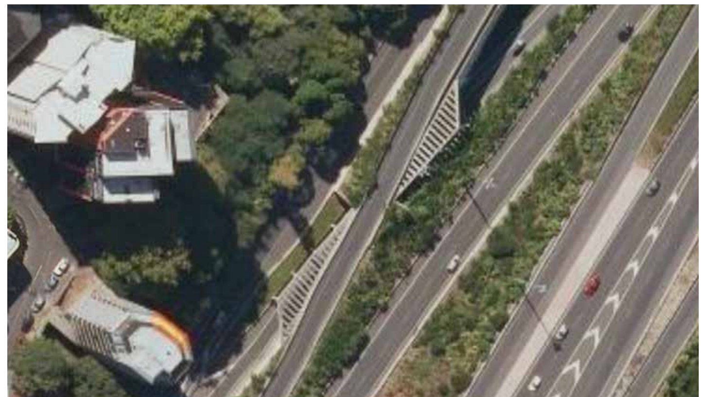
Figure 5.79: Grafton Gully structure similar to Bridge 27
