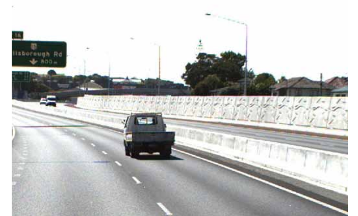
Photo 5.30: Concrete side barrier extended to act as noise wall
