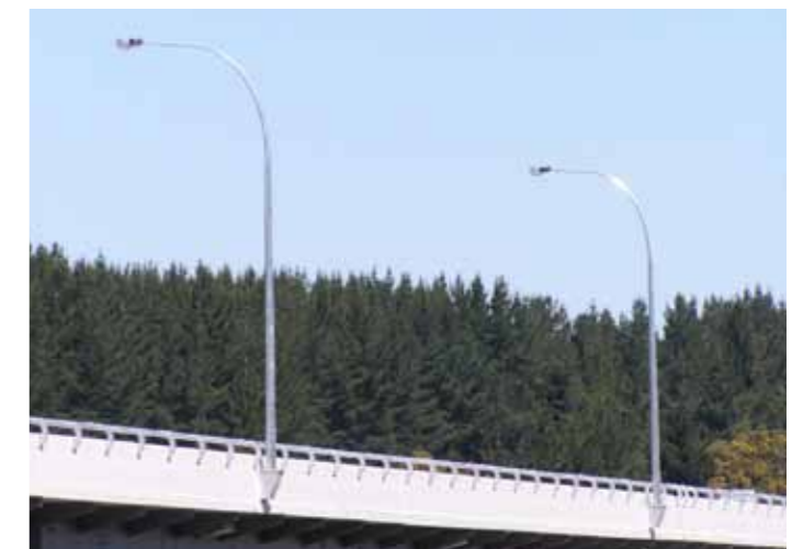
Photo 4.31: Light columns mounted to side of bridge
