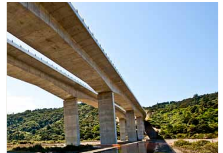
Photo 4.4: Elegant profile: Twin haunched girder bridges
