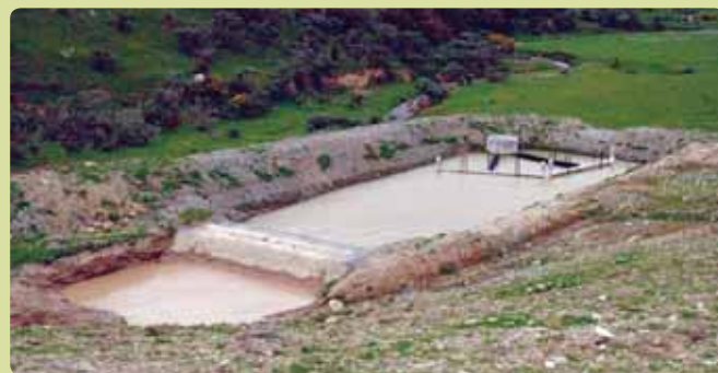
Example of a typical sediment control pond from Project West Wind - Photograph supplied courtesy of Meridian Energy Limited
