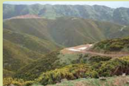
Example of a typical sediment control pond on a ridge in terrain similar to Transmission Gully from Project West Wind - Photograph supplied courtesy of Meridian Energy Limited
