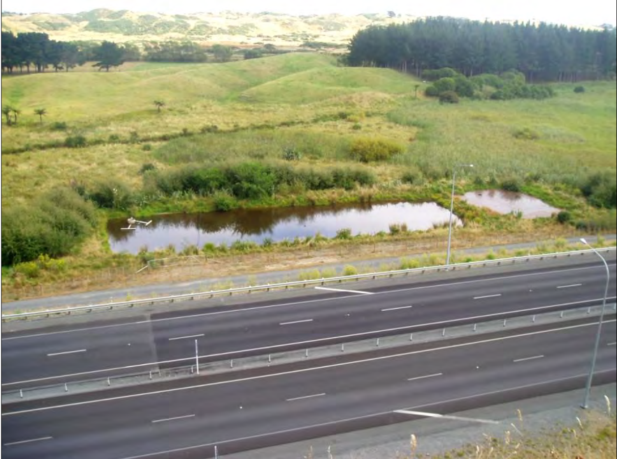
Photo 14 MacKays Crossing wetland with Raupo swamp centre and to the right (north), crack willow, swampy pasture and weedland to the left (south). Existing stormwater treatment pond in the foreground that will be incorporated into the new treatment pond structure.
