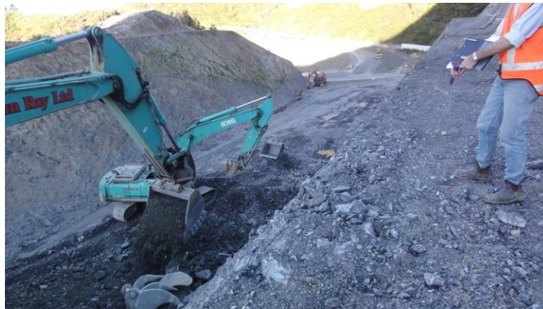
Photograph 2 – Earthworks at Muldoons Corner site
