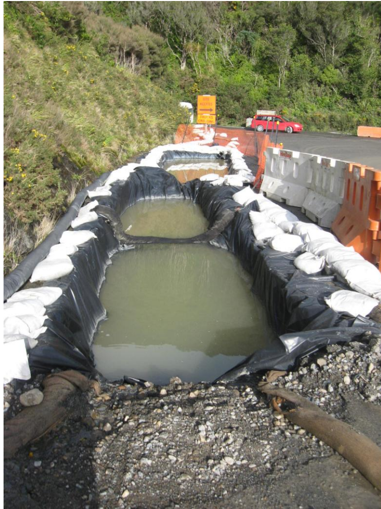
Photograph 3 – Sediment Pond at Muldoons Corner Site
