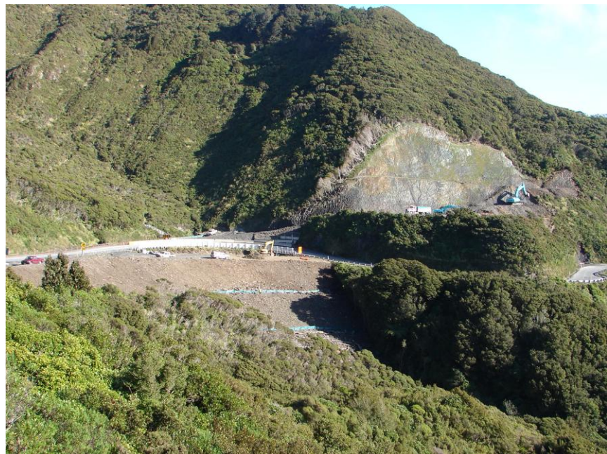
Photograph 1 – Earthworks construction at SH2 Muldoons Corner
