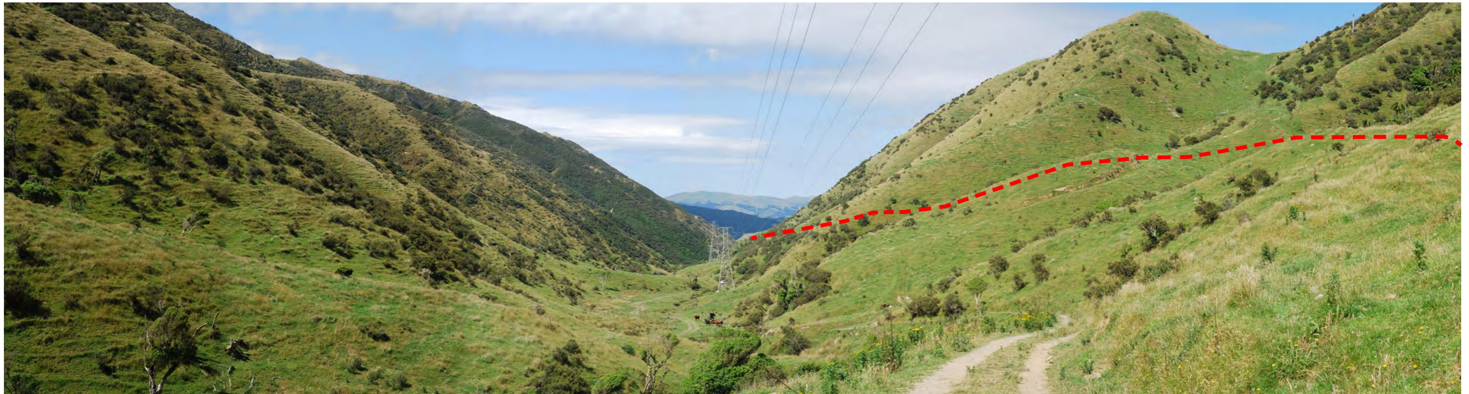
6) View to the south down Horokiri Stream Valley from below Wainui Saddle (Route Section 3)
