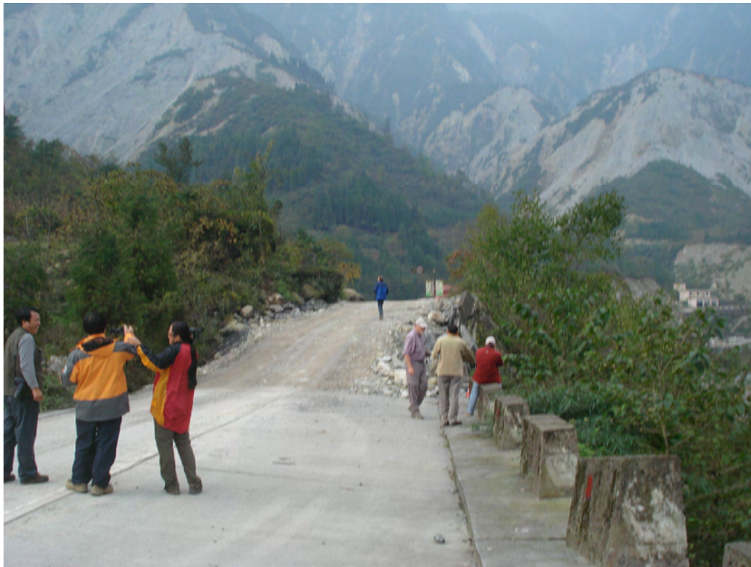
FAULT RUPTURE ACROSS EMBANKMENT, ACCESS RESTORED WITHIN DAYS AFTER THE 2008 WENCHUAN EARTHQUAKE, CHINA
