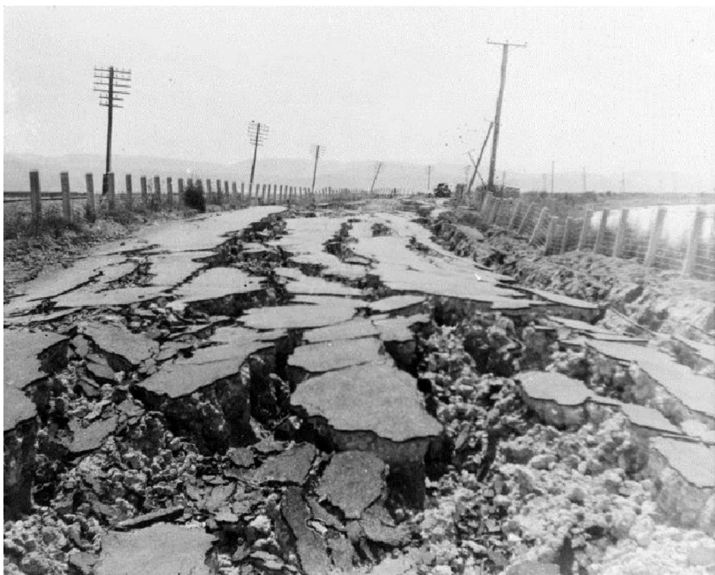
FAILURE OF ROAD EMBANKMENTS DUE TO LIQUEFACTION IN THE 1931 HAWKES BAY EARTHQUAKE
