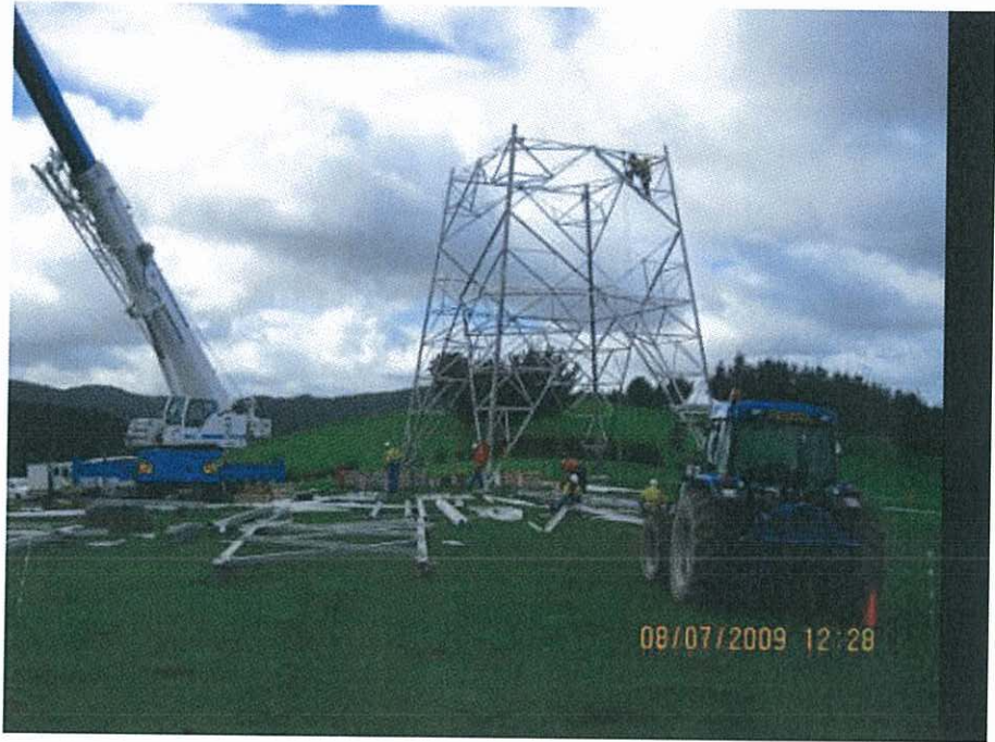
Photo 2: tower assembly and erection using crane techniques
