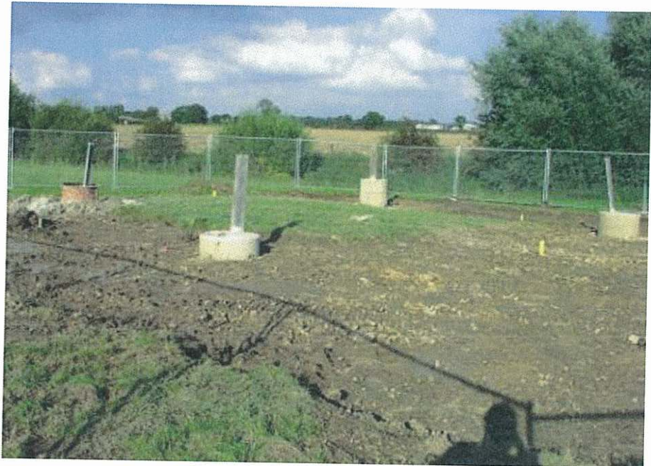
Photo 1: typical completed tower foundation
