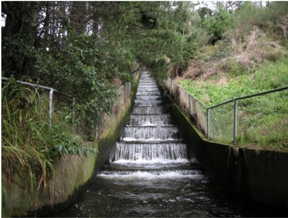
Figure 6.13: Like many of the waterways in the Kenepuru Stream catchment, parts of Cannons Creek have been significantly modified
