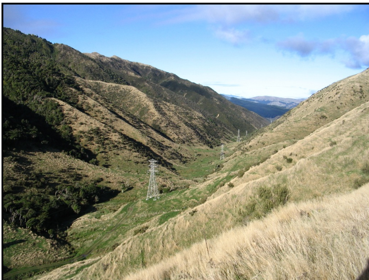
Figure 6.17: The existing PKK- TKR- A line looking southwards down the Horokiri Stream valley
