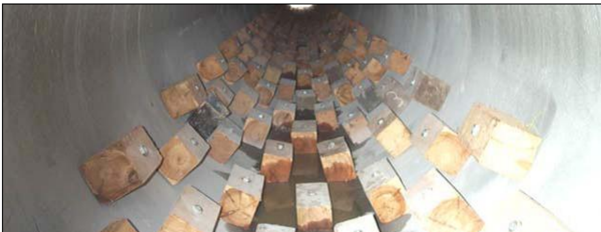
Figure 22.12: Wooden blocks bolted to culvert to improve fish passage
