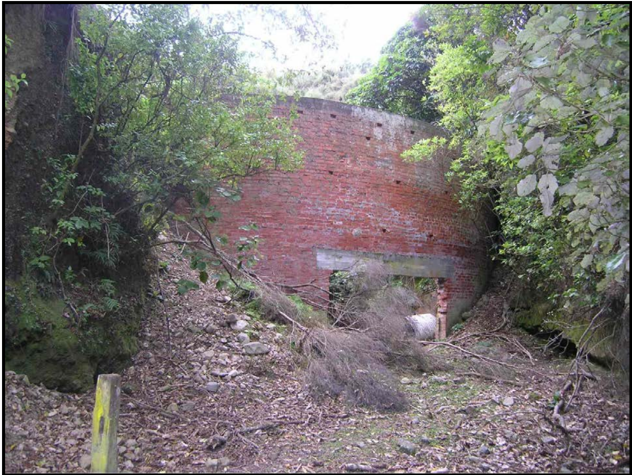
Figure 6.24: Brick fuel tank at the bottom of the Te Puka Valley, near MacKays Crossing
