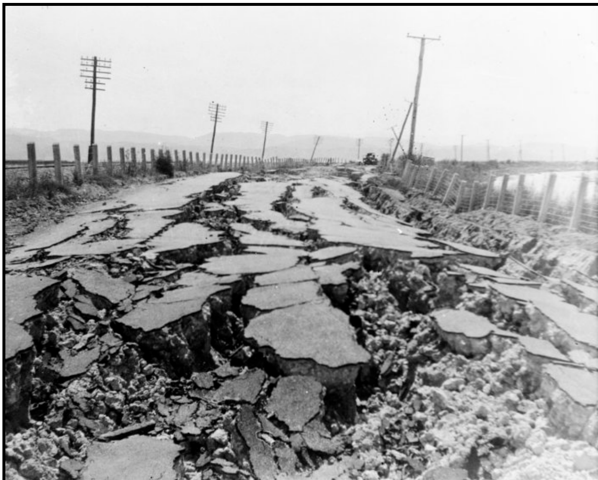
Figure 2.6: Damage to road from liquefaction and lateral spreading during the 1931 Napier earthquake
