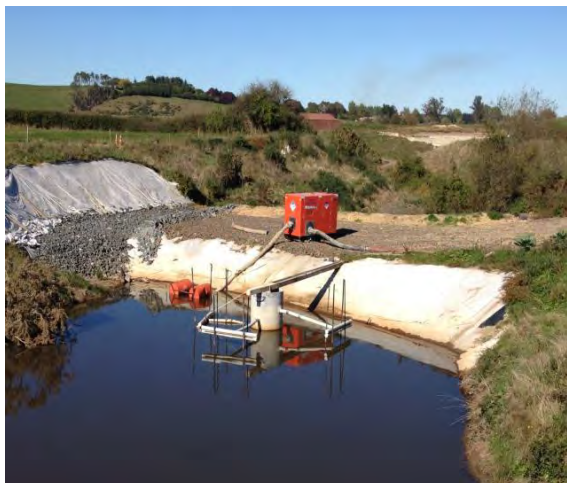
Sediment pond intake structure
