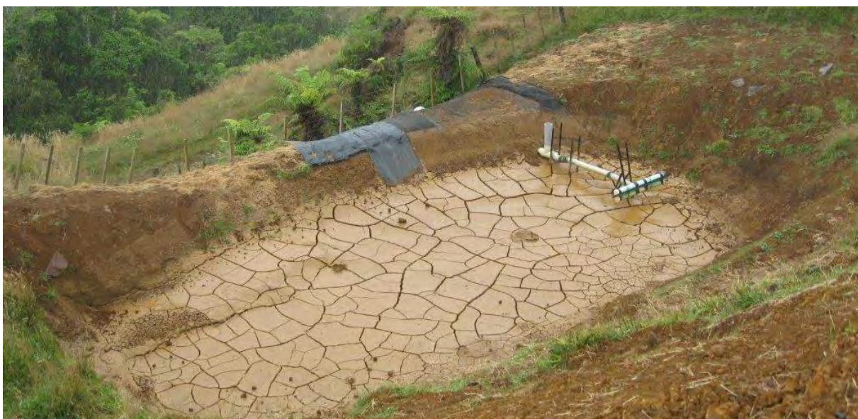
Decanting earth bund
