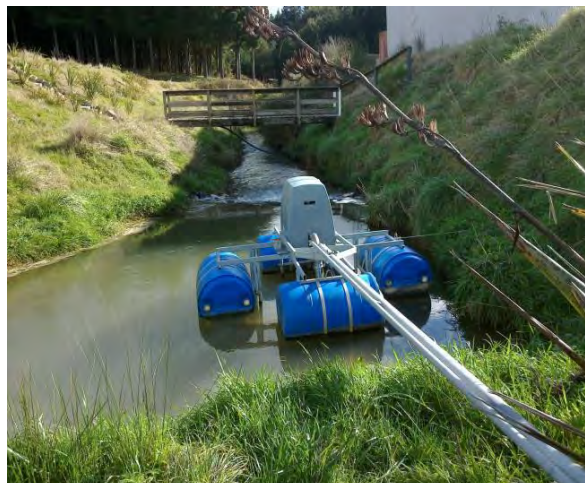
Surface water intake structure
