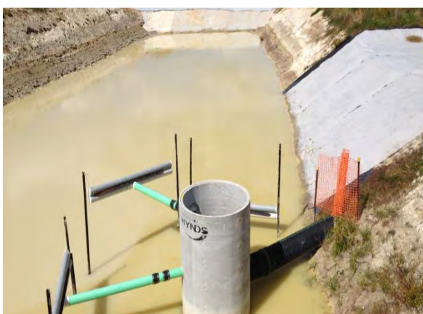
Sediment retention and treatment pond
