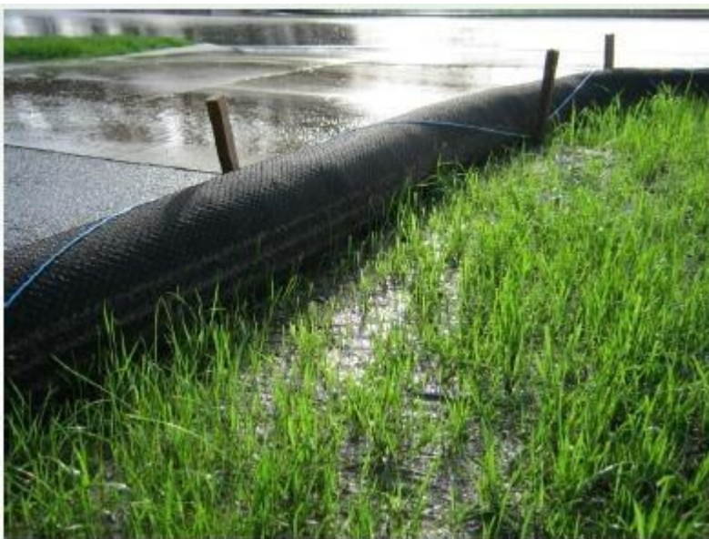
Figure 6.1. Silt or filter sock used as edge protection
