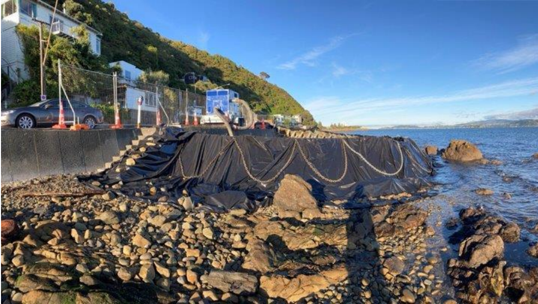
Figure 6.7. Example of wave barrier structure
