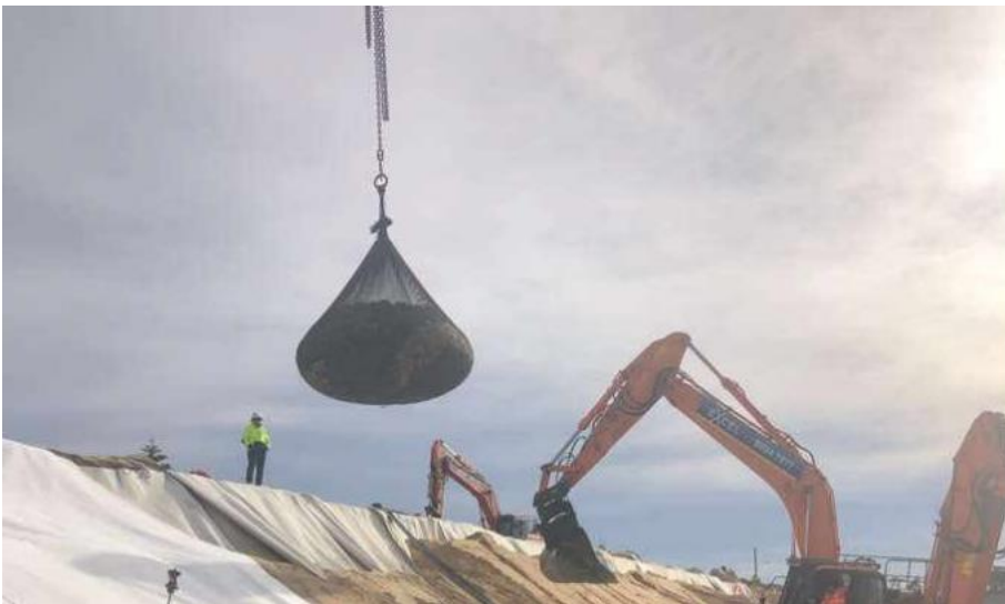
Figure 6.6. Example of a rock sock
