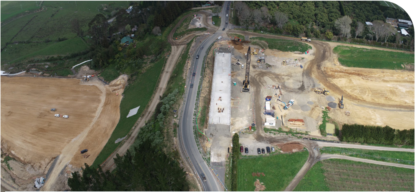
Wairoa Road Bridge
