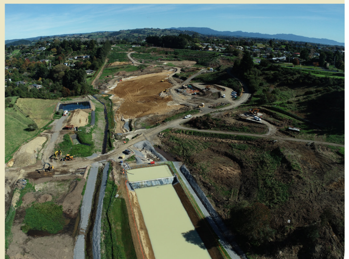
Aerial photo looking towards Bethlehem from the Smiths Farm area, April 2022
