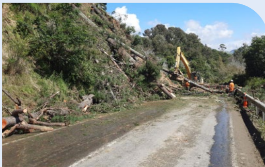
Removing trees from high-risk areas to help stabilise the slip faces
