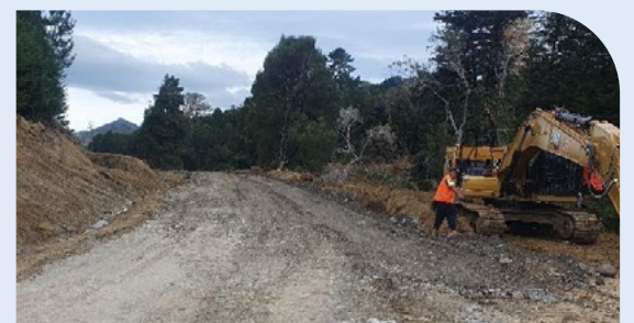
Progress on the temporary bypass in the Mangahauini Gorge - taken 13 March
