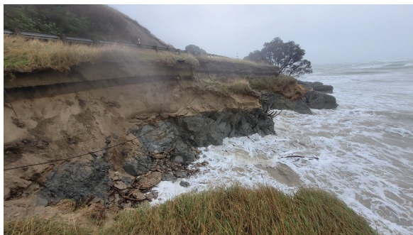
Coastal erosion at Turihaua Point in April 2022
